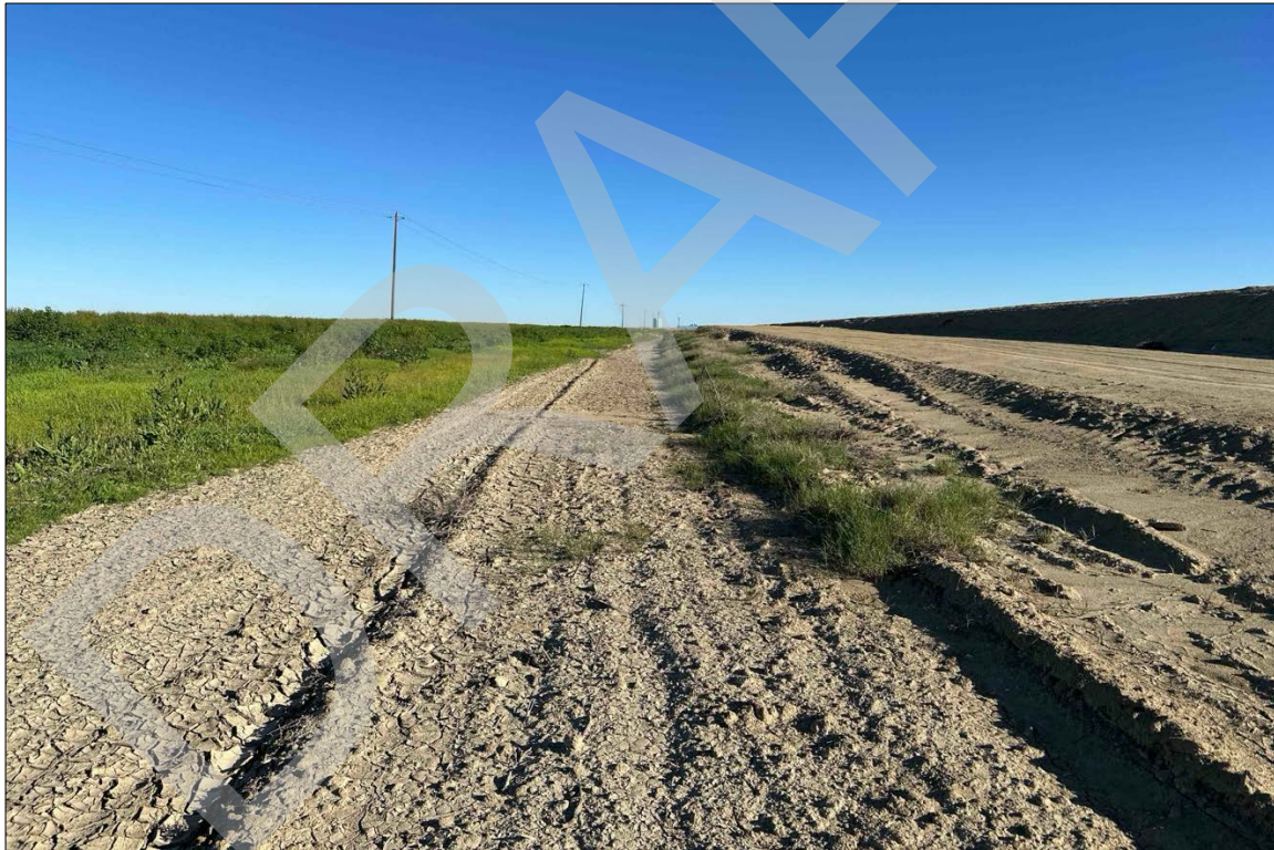
Figure 5. Photograph of the Project site perimeter, looking north, showing the California Aqueduct to the east (right).
