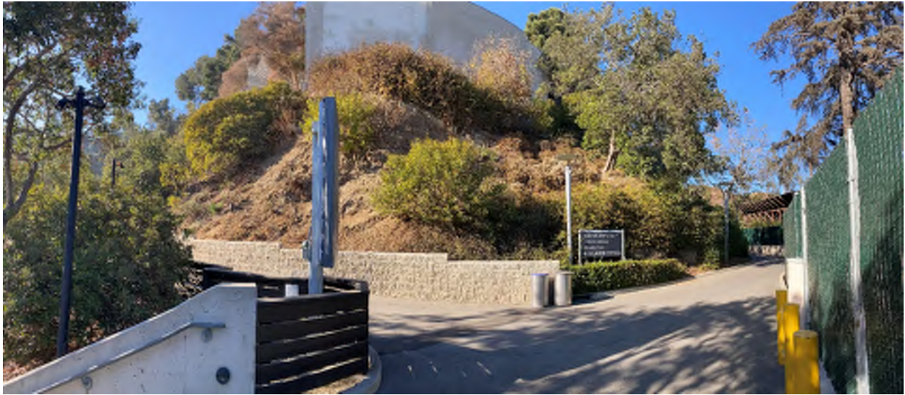
Figure 10: Existing Photo view 5 – Odin pathway view of concessions & restroom building at center top of photo. Proposed exit ramp located on the hillside. Existing block wall to be replaced as needed
