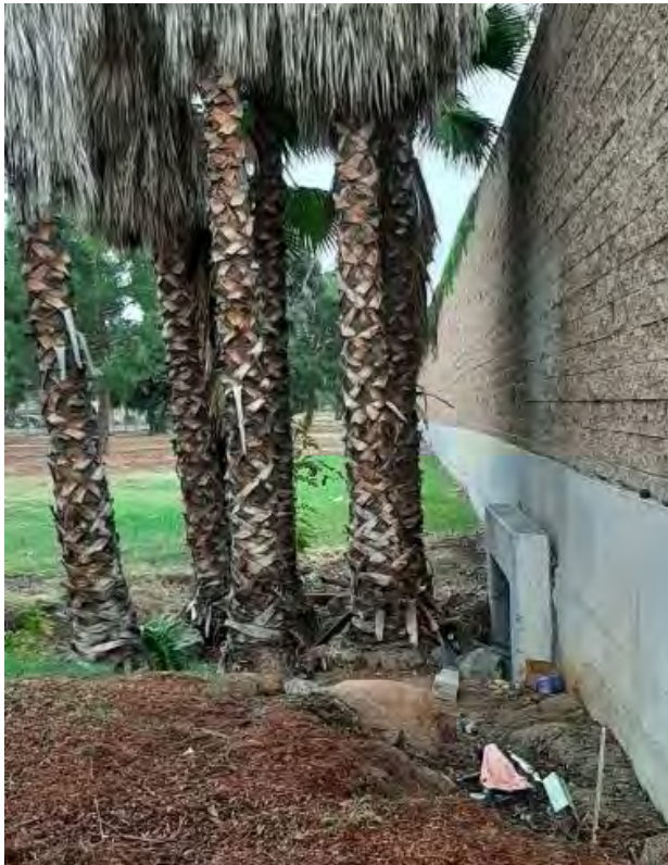
View at southern boundary looking west
