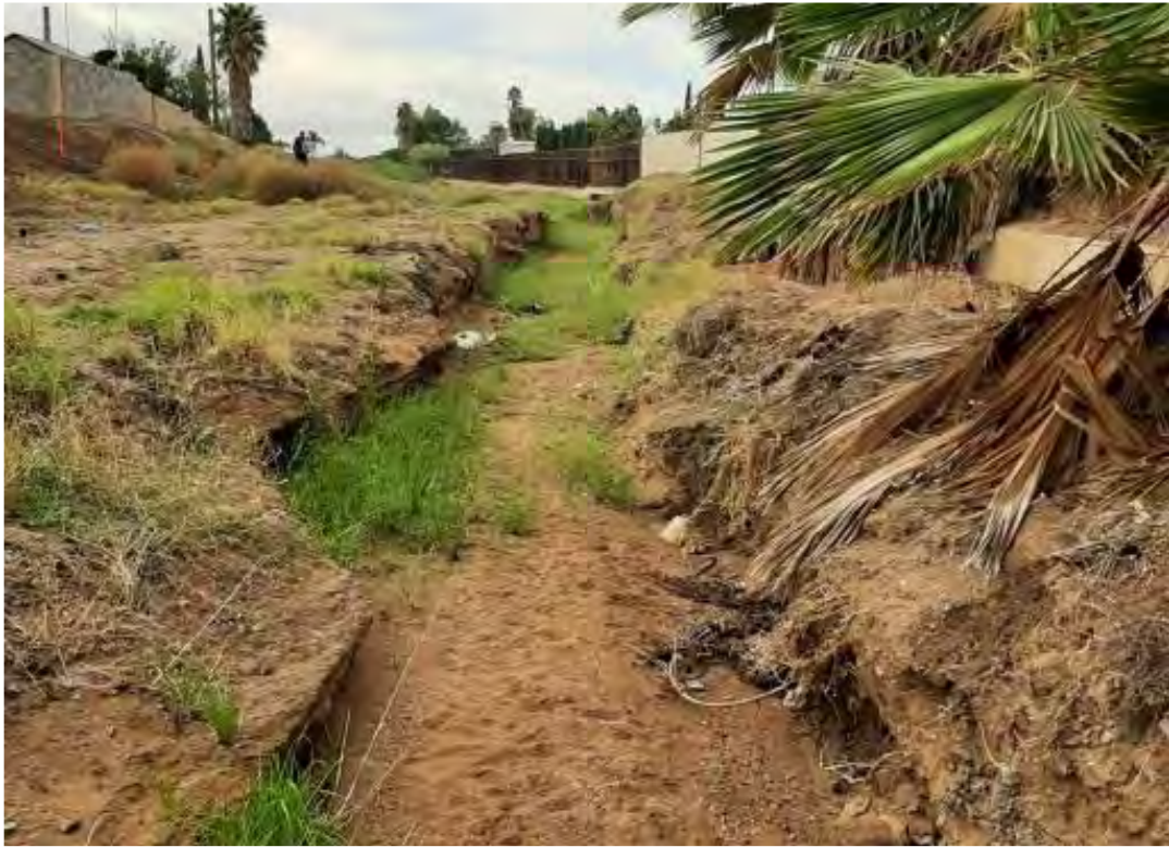
View of drainage channel looking south
