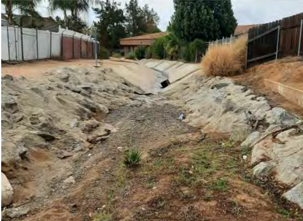
View of drainage channel looking south
