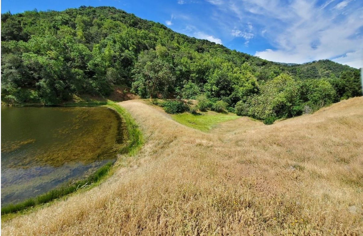
Photograph 1. The berm at the west end of RC-01, facing south.
