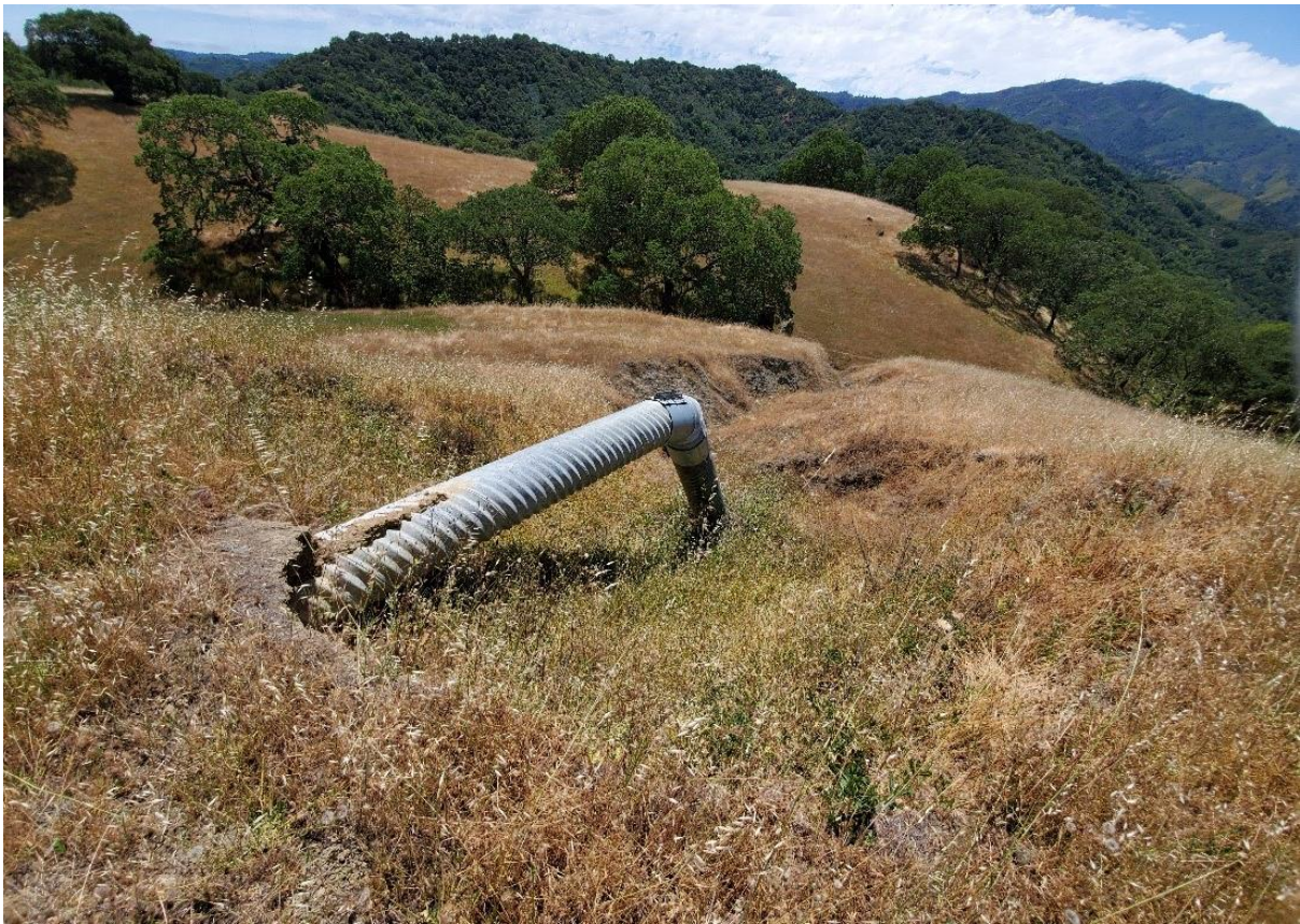
Photograph 4. The existing outfall at the west side of RC-07, facing southeast.
