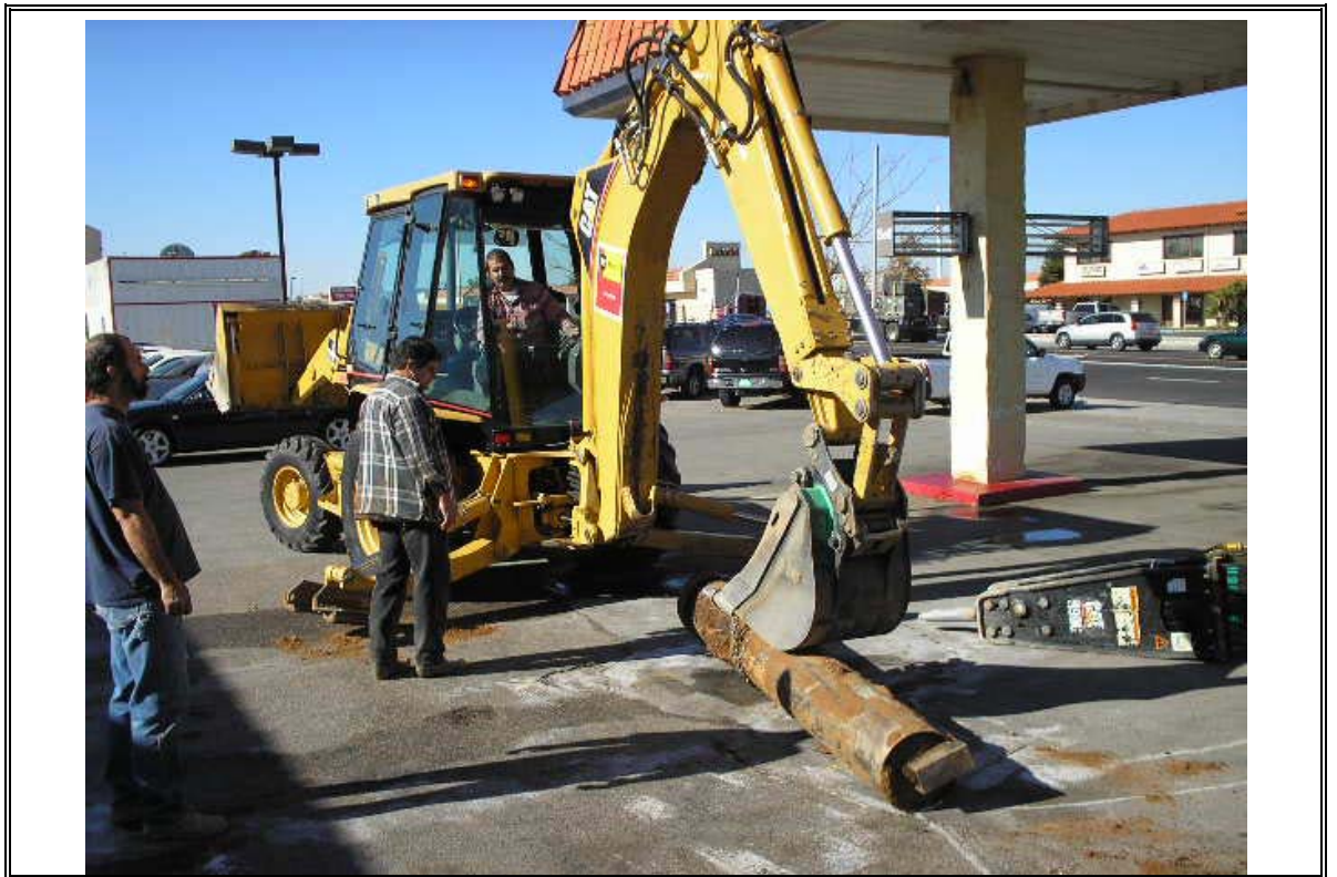
Photograph Number 5: Hydraulic lift cylinder removed from garage
