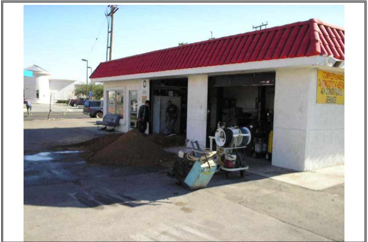
Photograph Number 3: Garage building following removal of hydraulic lift
