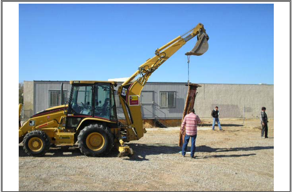
Photograph Number 9: Hydraulic left cylinder in southwest corner after removal
