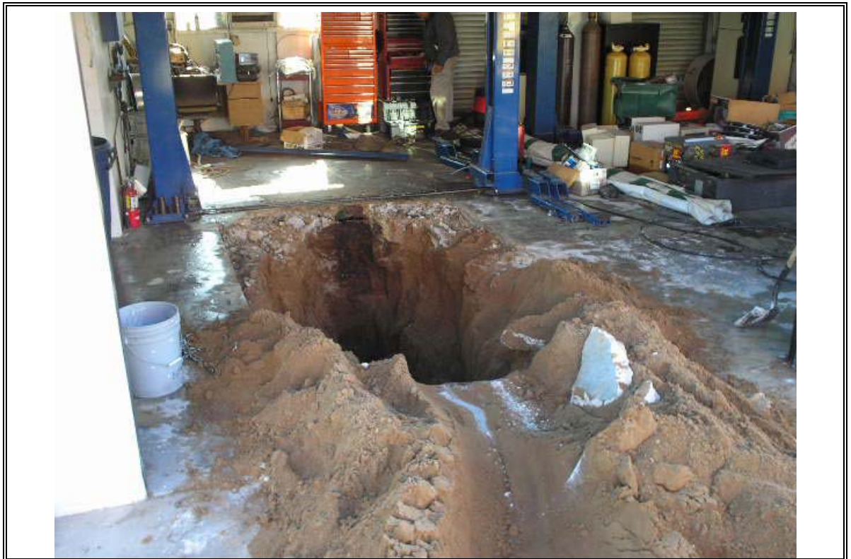
Photograph Number 4: Hydraulic lift removal excavation in Garage
