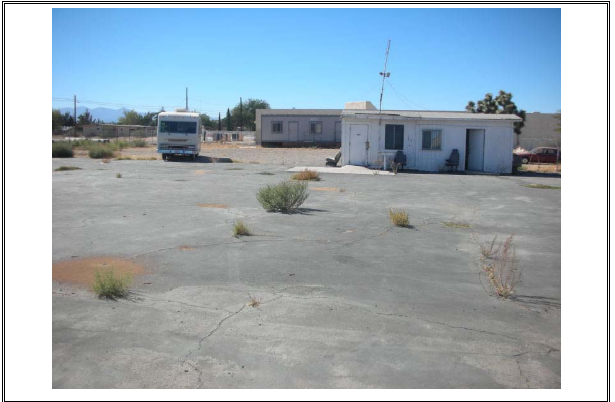
Photograph Number 6: View west of buildings on the southern portion of the Site. Hydraulic lift is behind portable office in the background, southwestern corner of Site.
