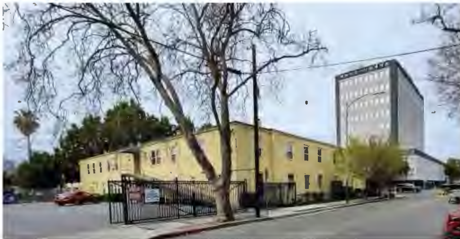
Photograph 4 610-650 E. Santa Clara Street View: Southeast corner, showing the rear and east facades Date and Camera orientation: March 14, 2021 Facing-Northwest
