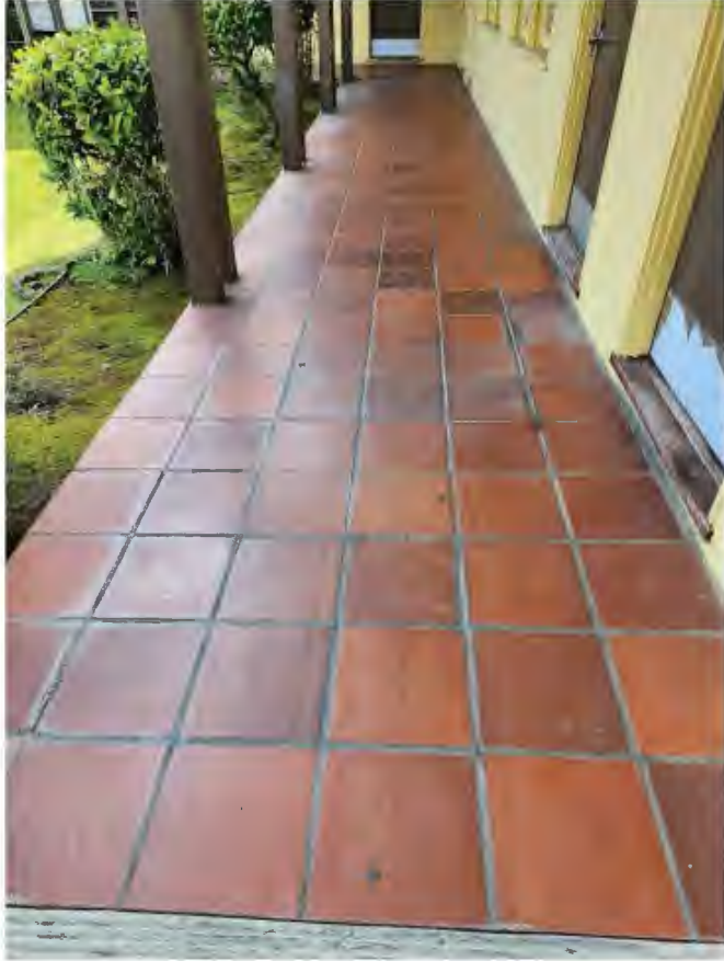
Photograph 8 610-650 E. Santa Clara Street
