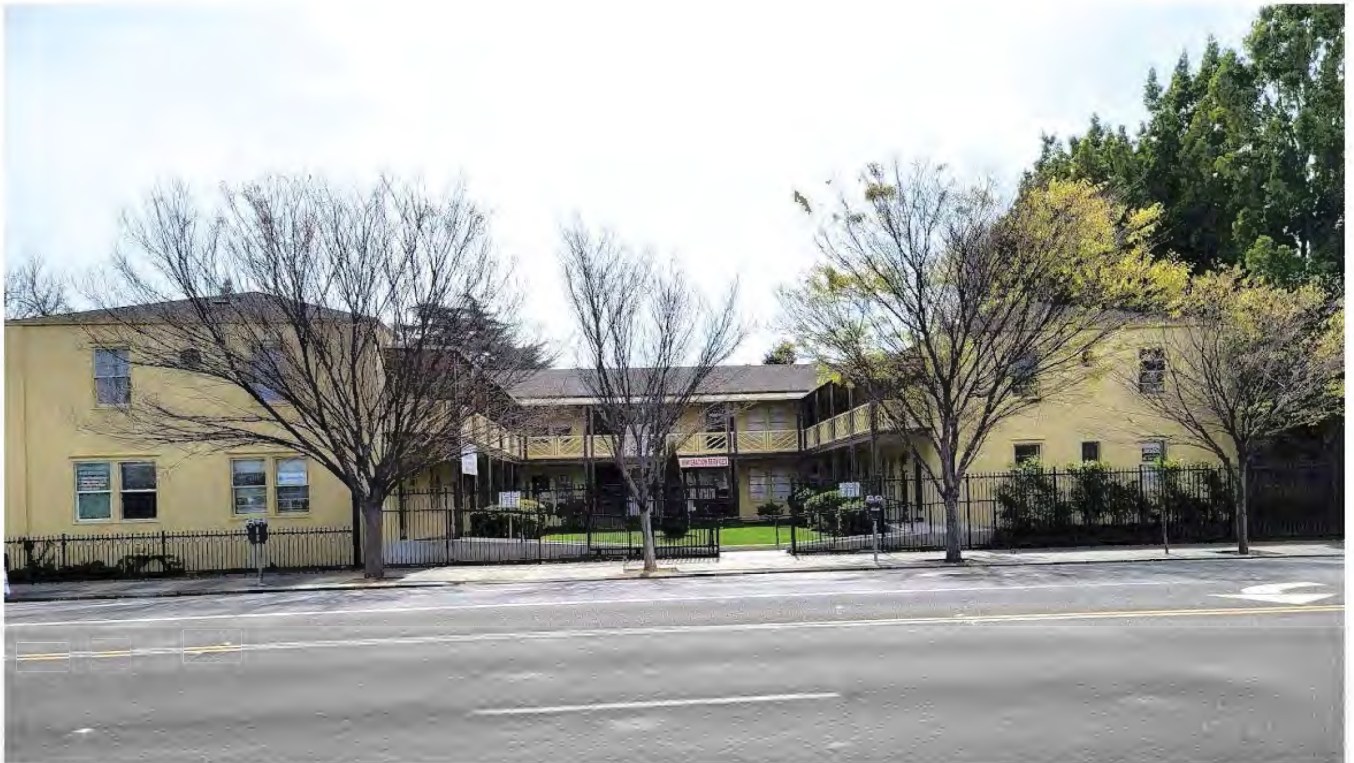
Photograph 1 610-650 E. Santa Clara Street View: Front façade of the “U” shaped, two-story building Date and Camera orientation: March 14, 2021 Facing-South
