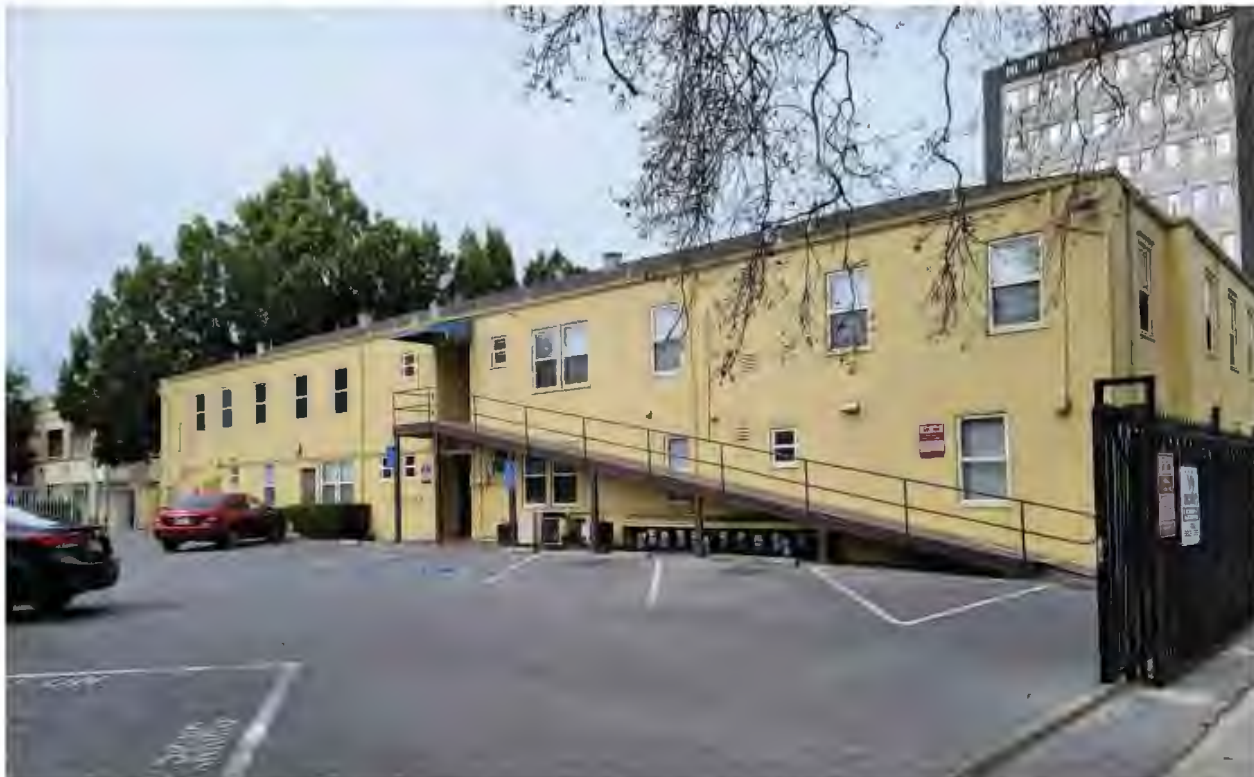
Photograph 5 610-650E. Santa Clara Street View: Rear (South) Façade with ramp Date and Camera orientation: March 14, 2021 Facing-North
