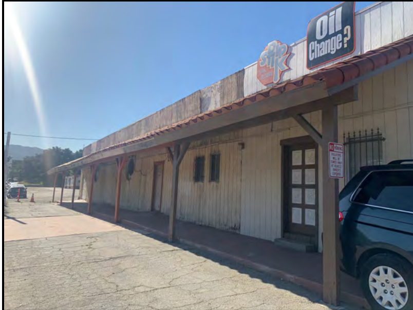
Figure 10: Overview of a 1940s addition to the home to create a large frontage on Newhall Avenue (facing southwest).
