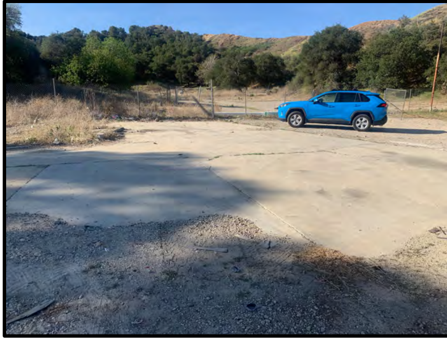
Figure 13: Overview of Foundation 1.
