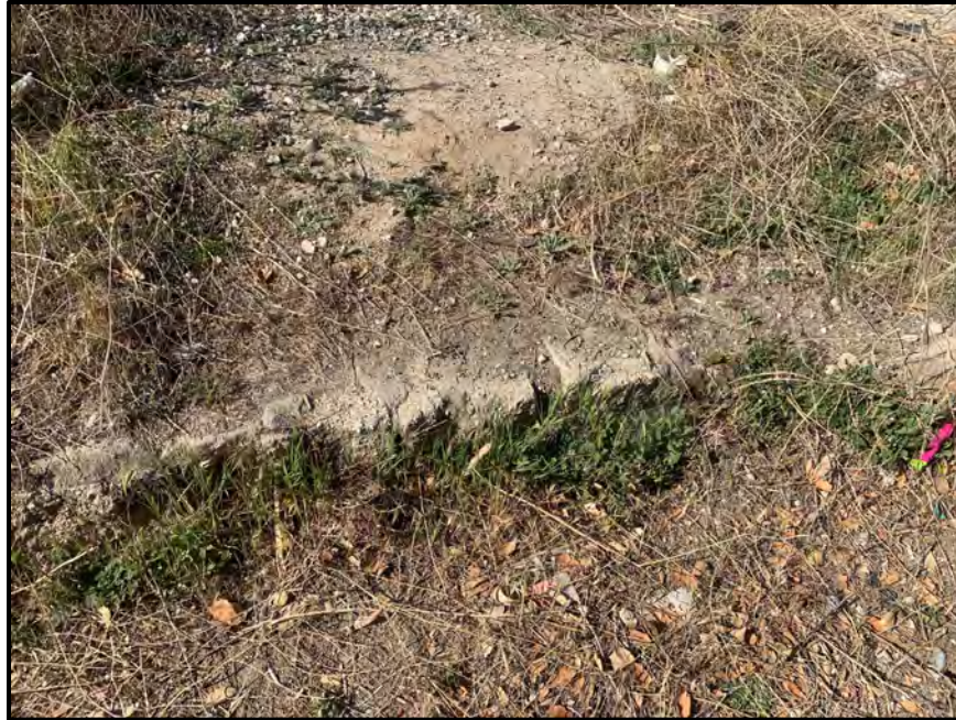
Figure 11: Overview of Wall 1.
