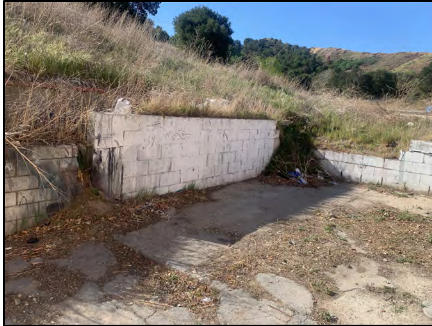
Figure 17: Overview of Foundation 5 with Wall 3.
