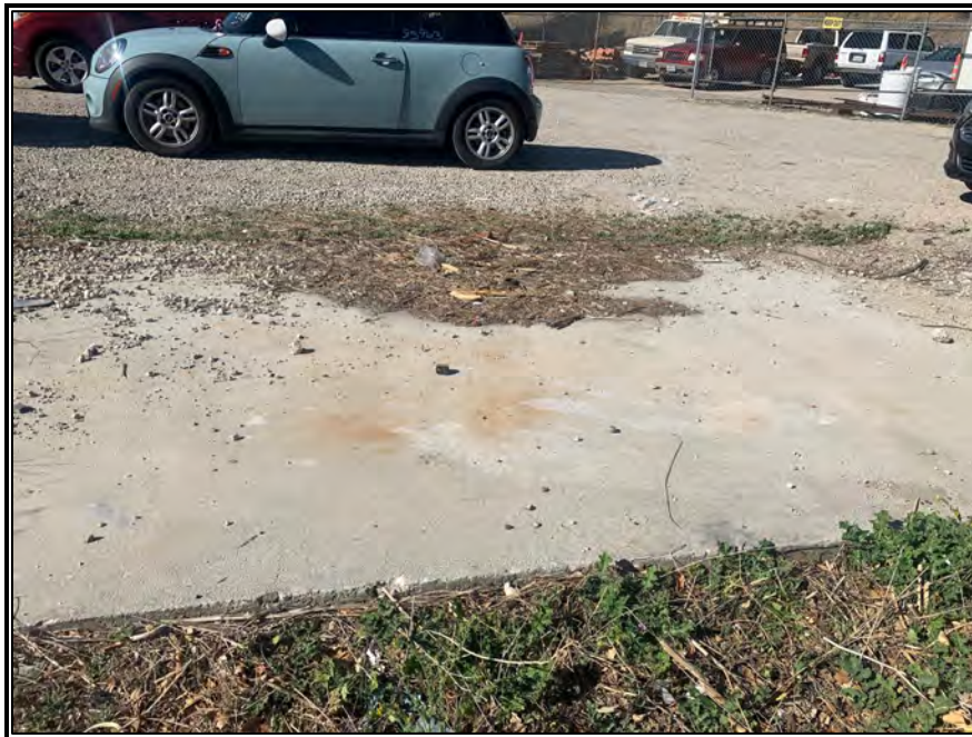
Figure 14: Overview of Foundation 2.
