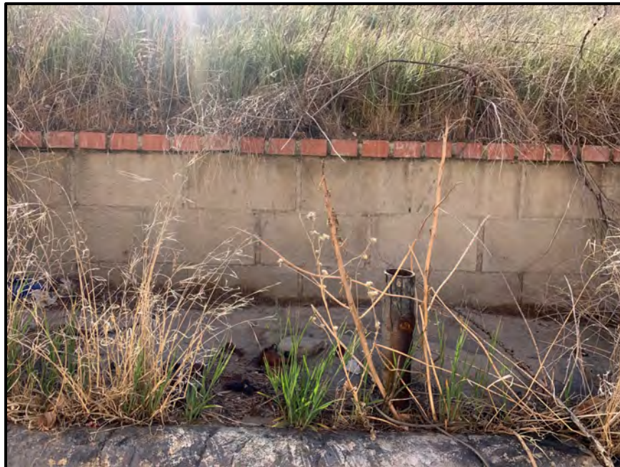
Figure 12: Overview of Wall 2.
