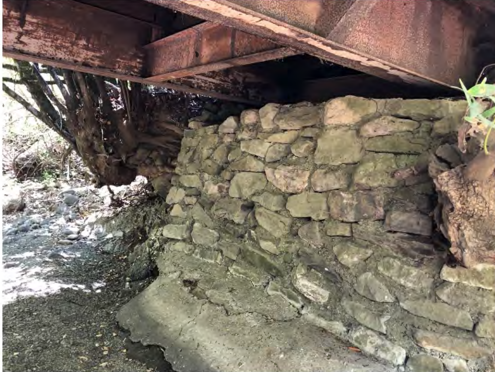
Photo 3. Underside of existing bridge showing structural foundation on west bank.
