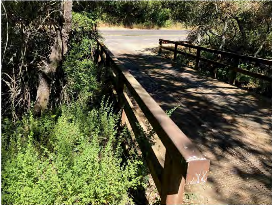
Photo 1. View of existing bridge looking towards Mt. Veeder Road.
