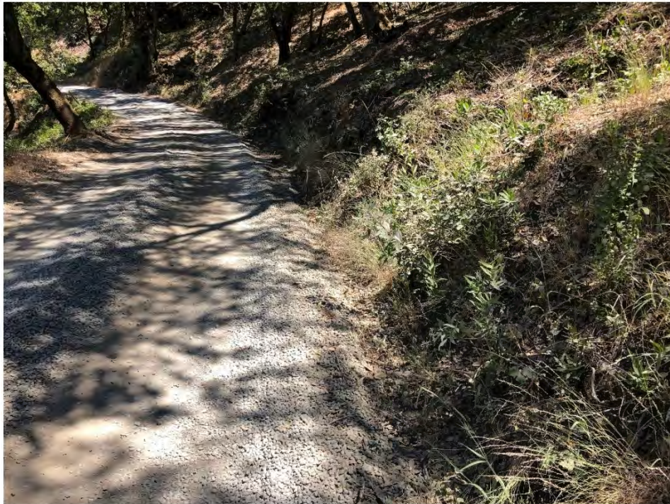
Photo 4. View of existing driveway with roadside drainage ditch.
