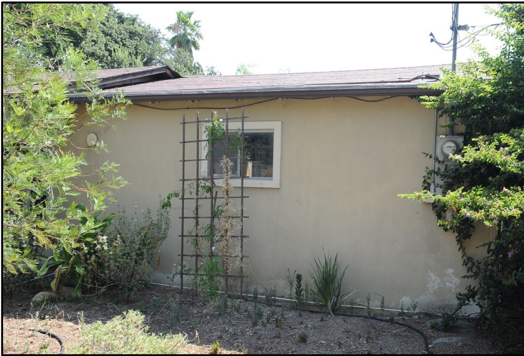
PHOTOGRAPH 3 West Elevation of Garage
