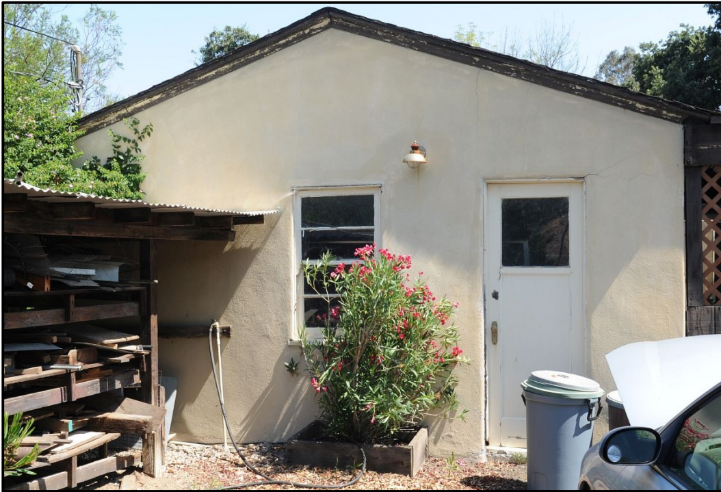
PHOTOGRAPH 9 South Elevation (Garage)
