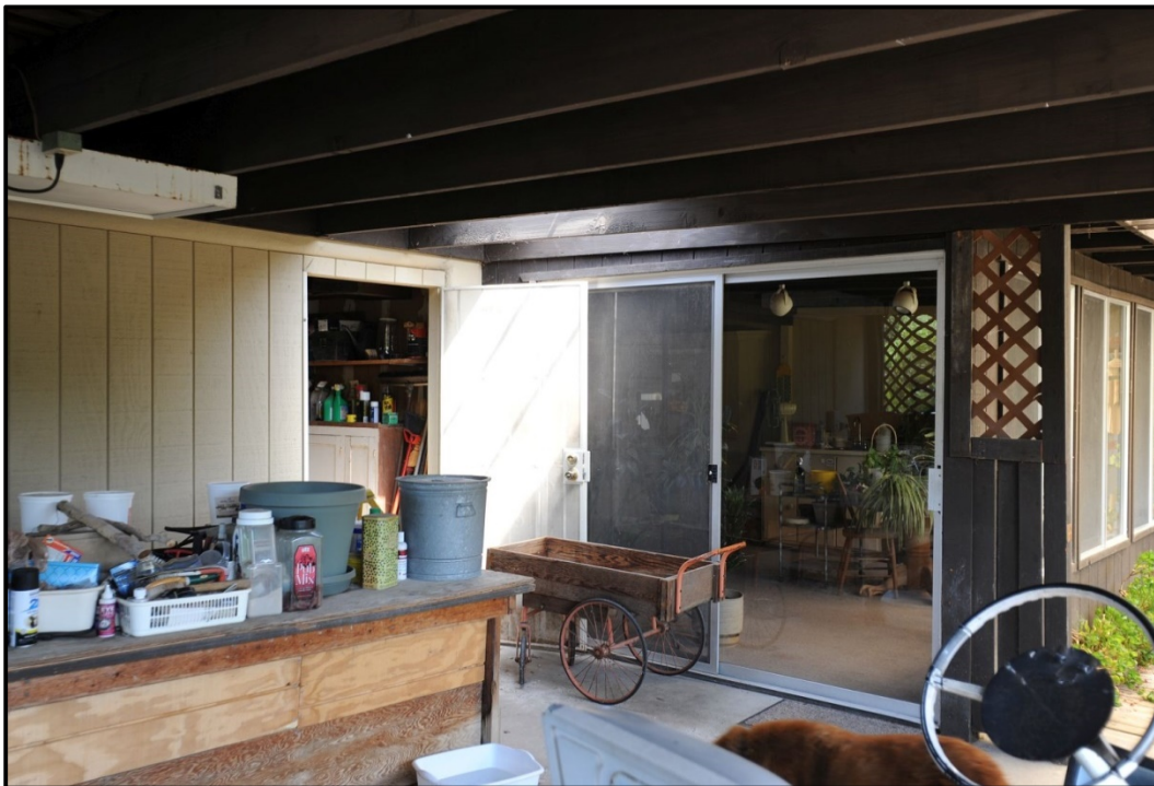
PHOTOGRAPH 8 East Elevation, Addition and Garage
