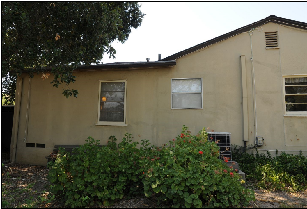
PHOTOGRAPH 5 North Elevation, East Half
