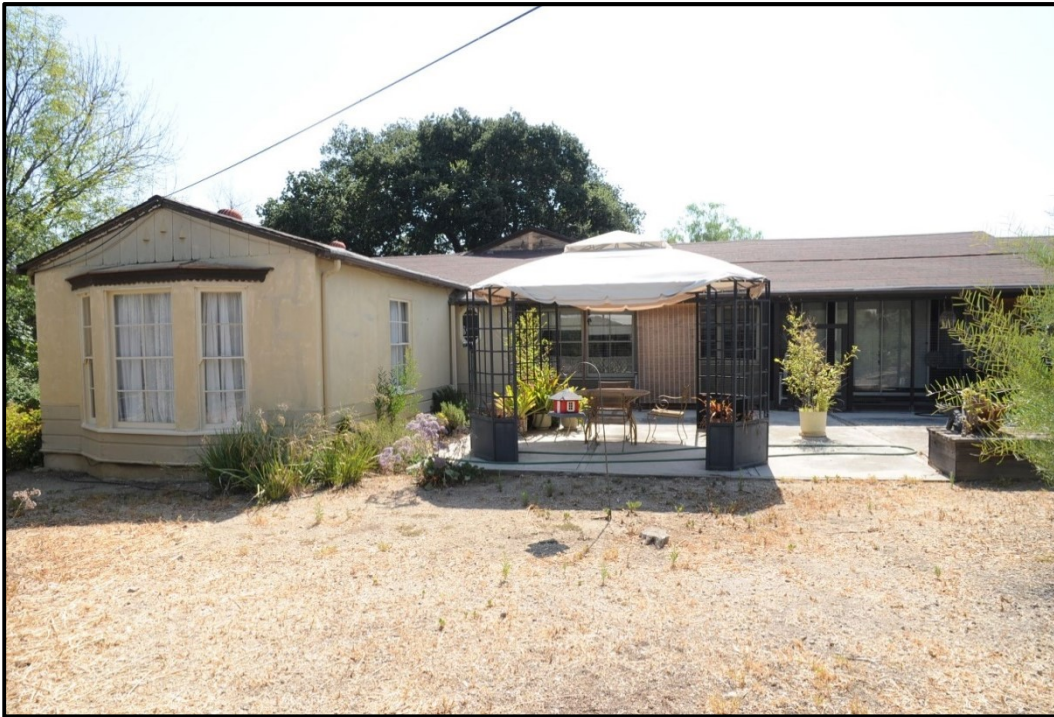
PHOTOGRAPH 1 View of Façade (West Elevation)
