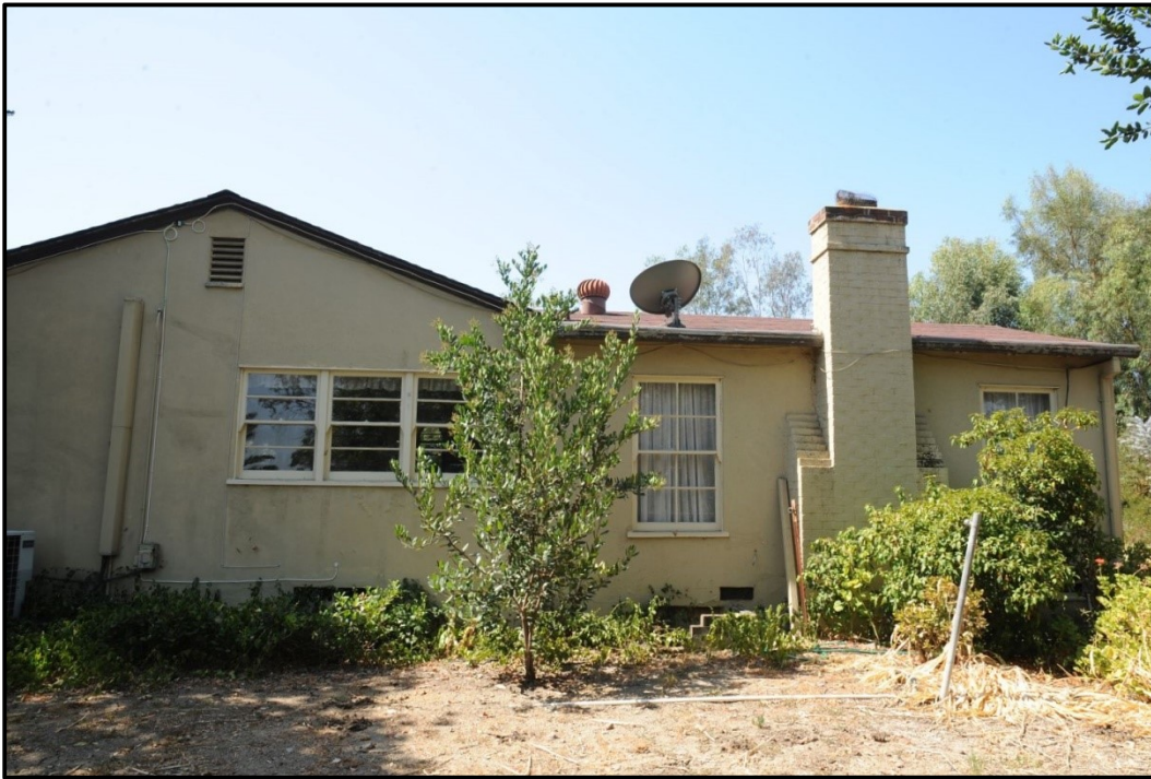
PHOTOGRAPH 4 North Elevation, West Half
