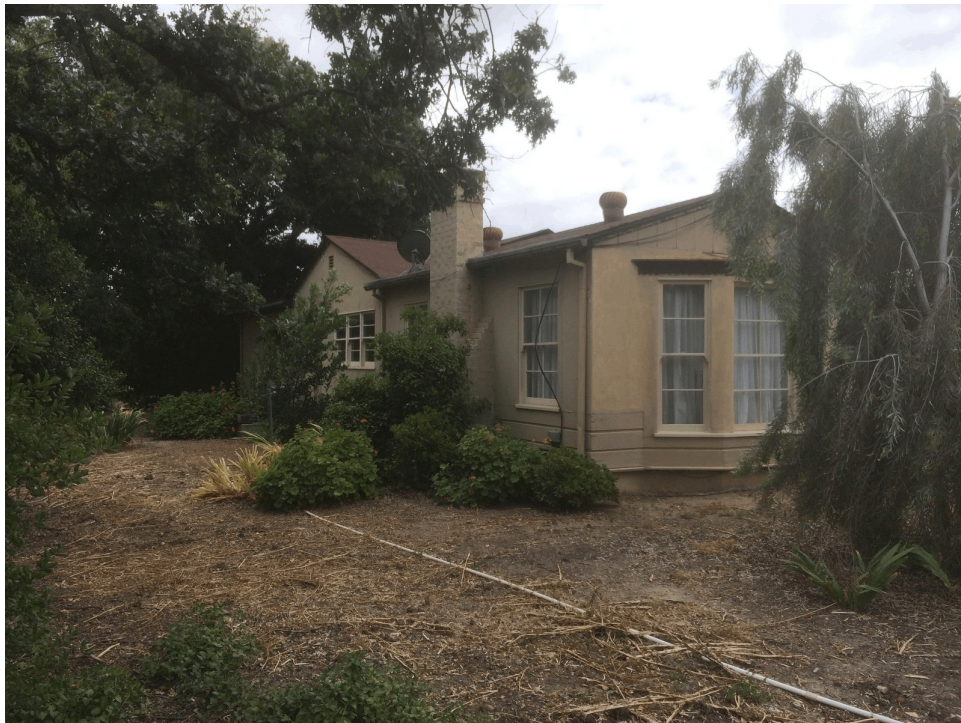
Photograph 6: View of the occupied Property residence looking southeastward
