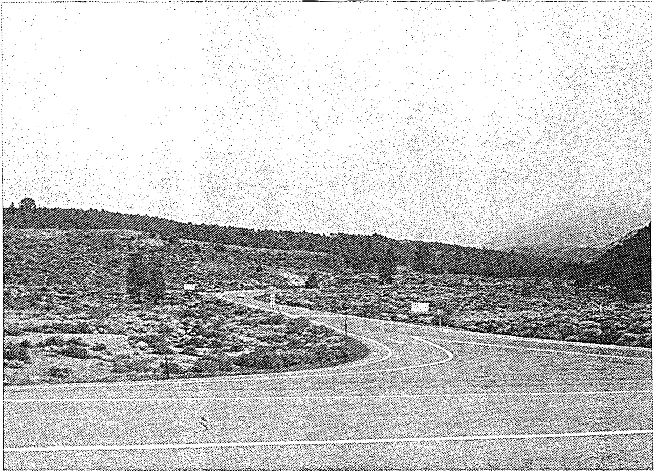
Plate F: View from north side of U.S. 395 looking south showing the U.S. 395-Tioga Pass view corridor.
