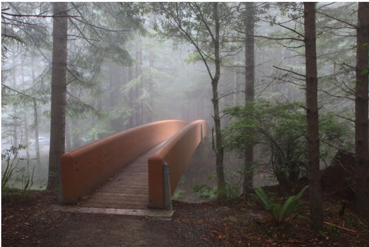
Pedestrian bridge across road in Redwood National Park. See http://www.redwoodhikes.com/RNP/LBJ.html
