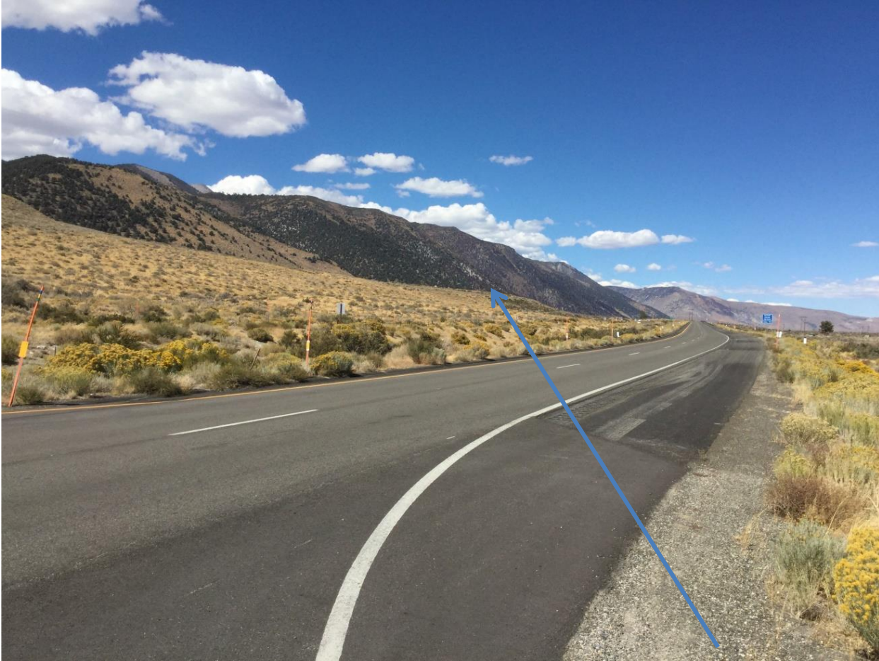
EXHIBIT 5.12-3. Existing Site View from US 395 at Picnic Grounds Rd.
