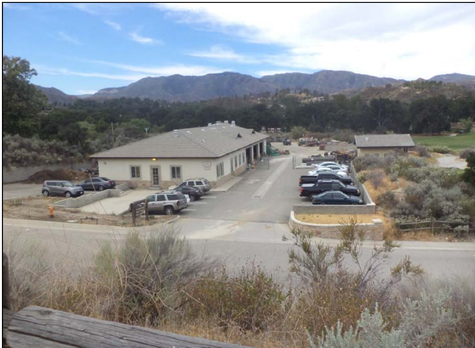
Photo 22: View of the maintenance building associated with the larger Sand Canyon Country Club property located across Robinson Ranch Road to the south.
