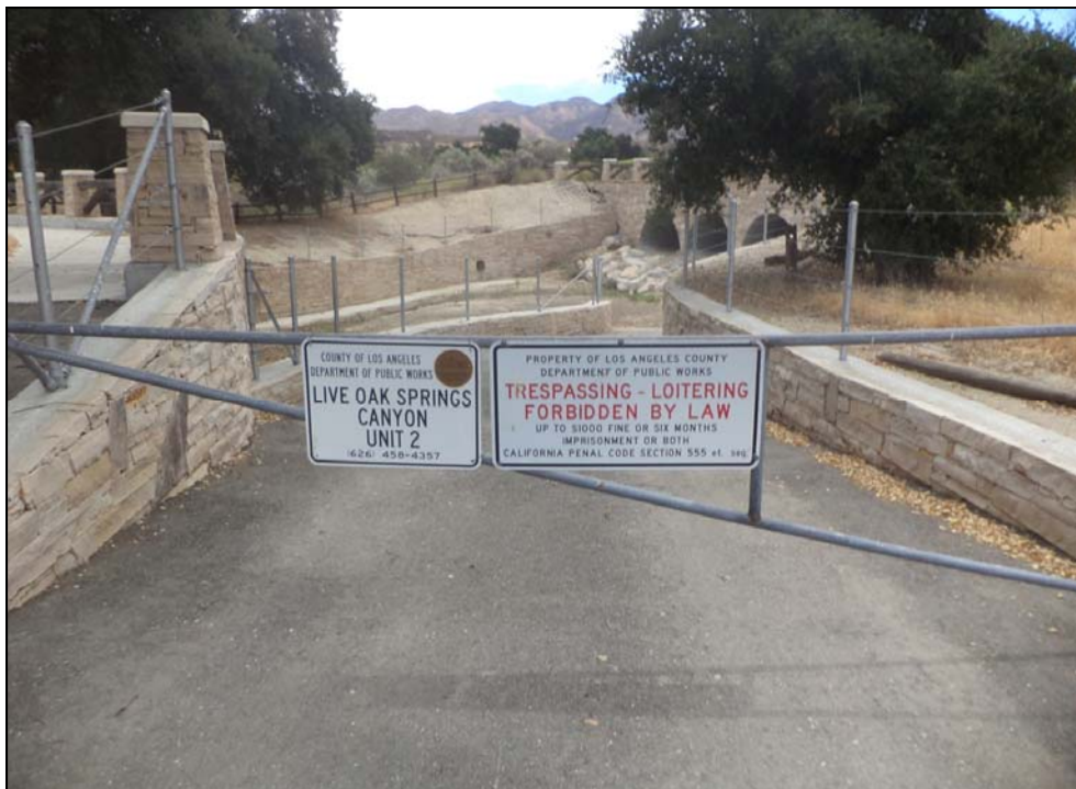
Photo 20: View of the Los Angeles County Department of Public Works flood control easement on the southwest corner of the subject property.
