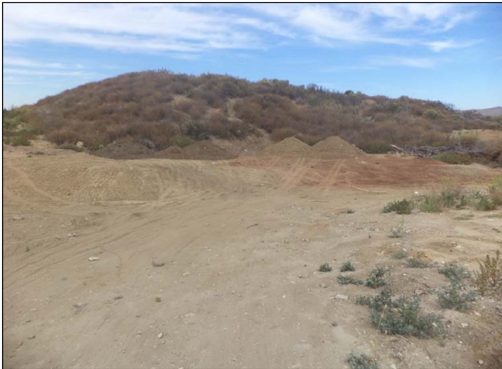
Photo 10: View of evidence of earth-moving activity near the southeastern portion of the subject property.
