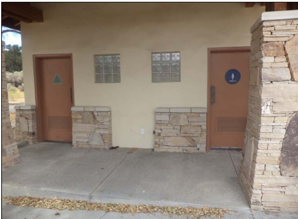
Photo 18: View of the entrance to the restroom structure.
