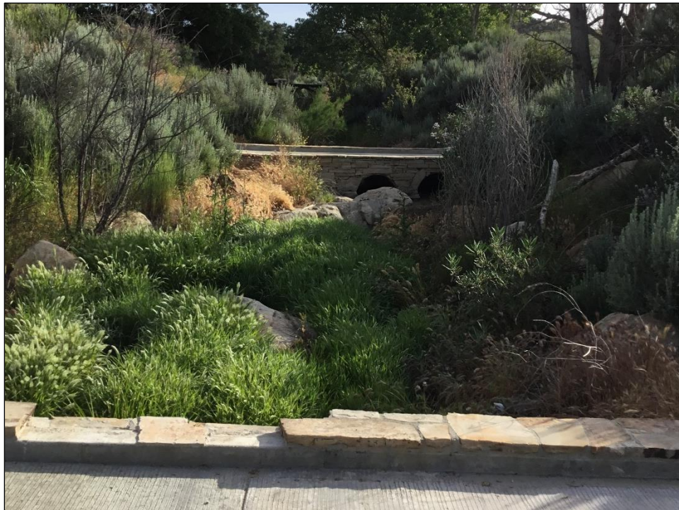
Figure 11. Overview of drainage area looking from pedestrian bridge in central of propose detention basin location; View facing north.
