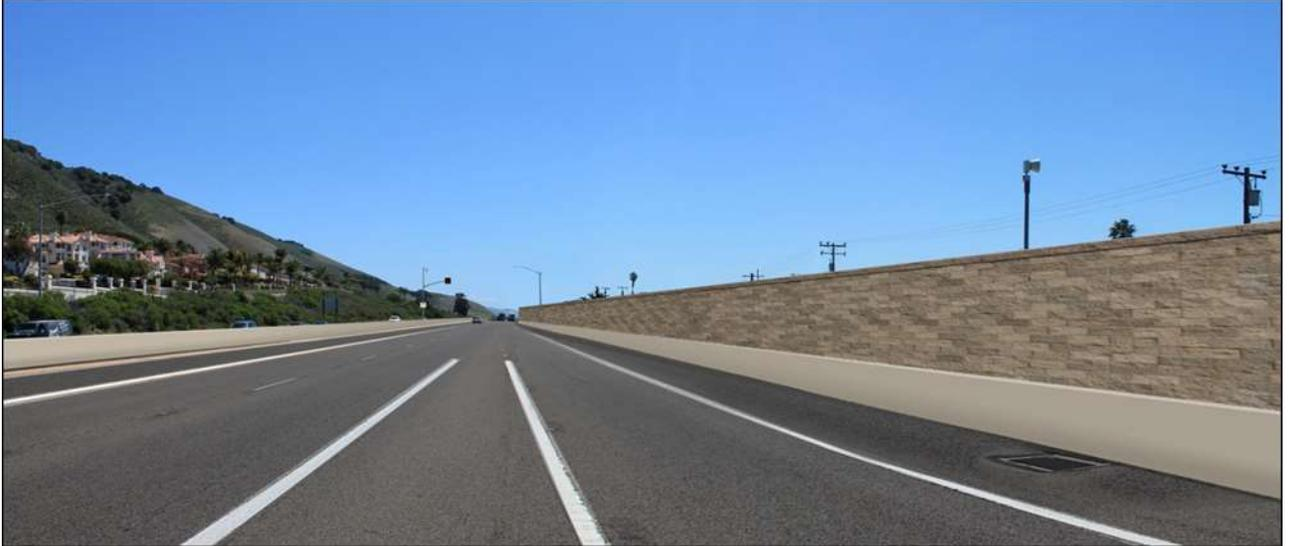
If it were constructed, an 8-foot-tall soundwall would be placed along the edge of the southbound freeway shoulder, possibly fronted by a concrete safety barrier. Existing vegetation between US 101 and Shell Beach Road would be removed to accommodate the part-time travel lane, and the existing concrete barrier in the median would be replaced with a taller style.
