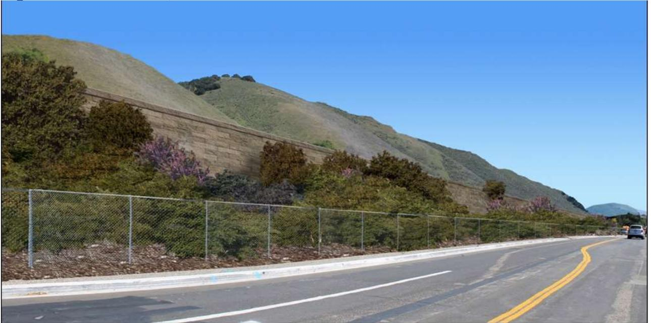
In this location, a 10-foot-tall soundwall is being considered for construction along the edge of the southbound US 101 outside shoulder. Existing vegetation between US 101 and Shell Beach Road would be removed to construct the wall and rebuild the associated slope.
