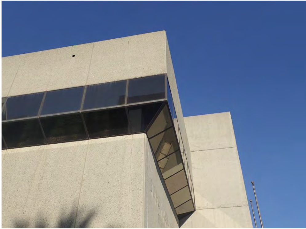
Detail view at southwest corner of building, viewed facing east.
