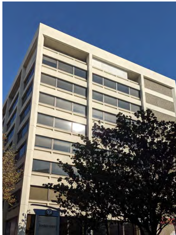
View of upper west elevation from San Fernando Street.
