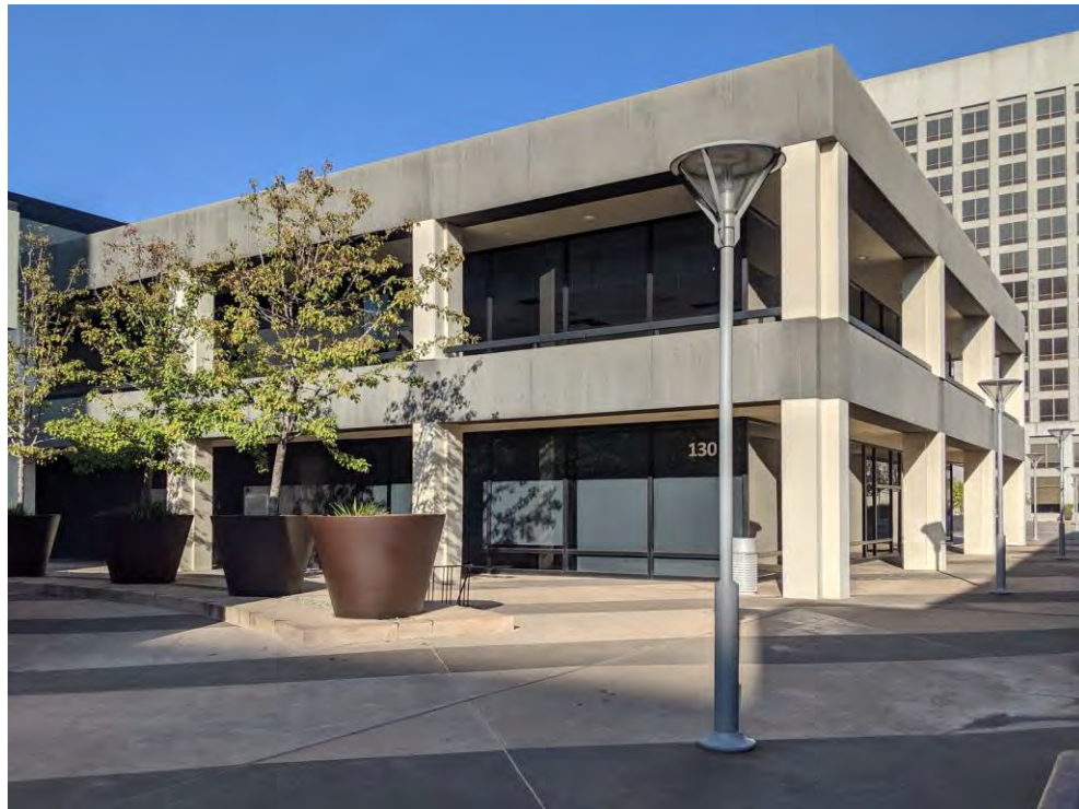
West elevation of 130 Almaden Blvd. pavilion viewed facing northeast.
