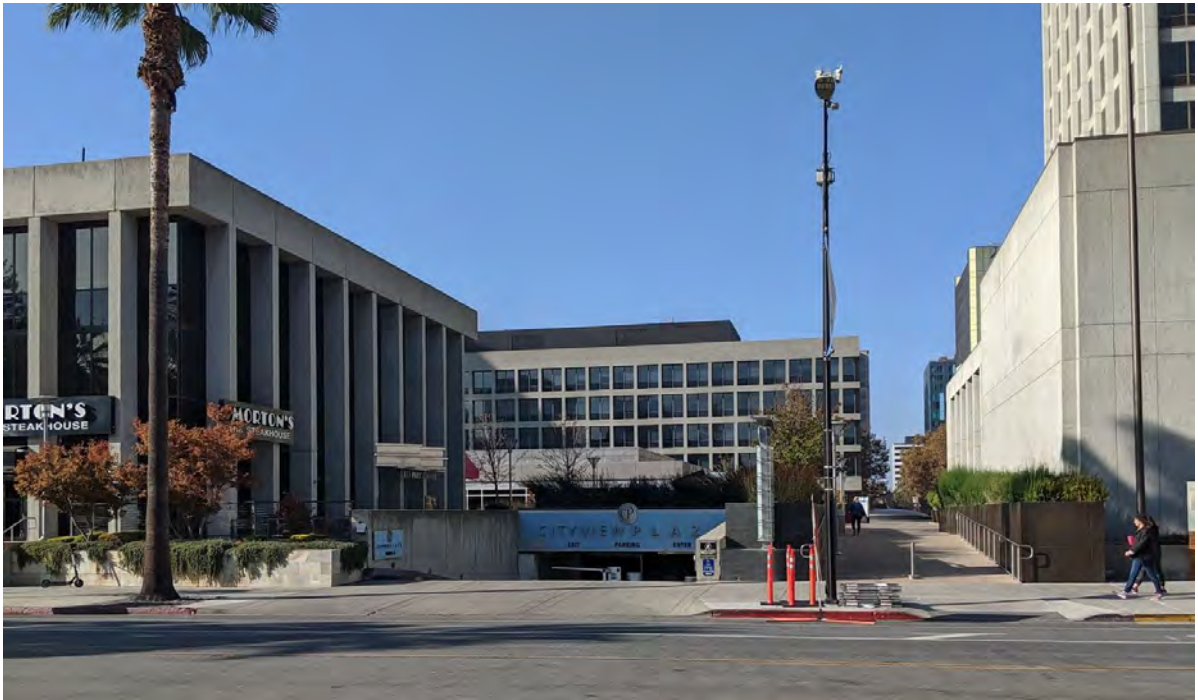
East elevation at garage entry, viewed facing north.
