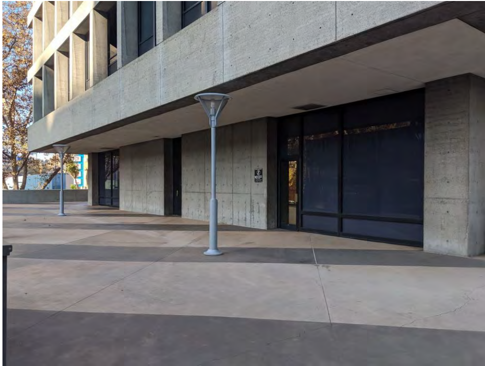
Plaza level of Landmark office building at west end, facing north.
