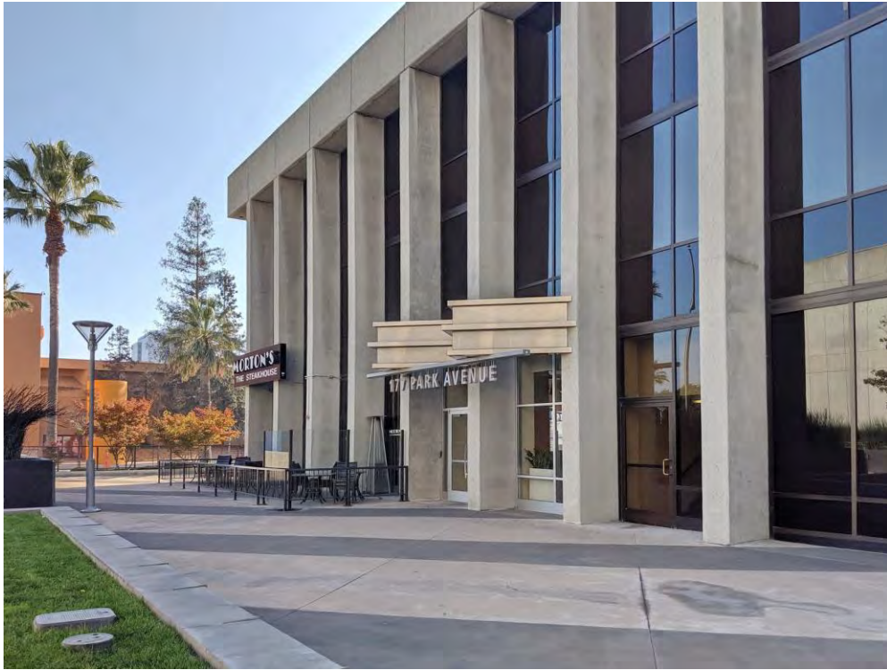
Entry off plaza at east elevation, viewed facing south.
