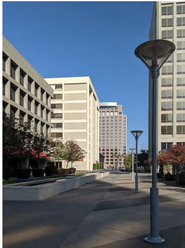
Plaza deck south of Landmark office building, facing east.
