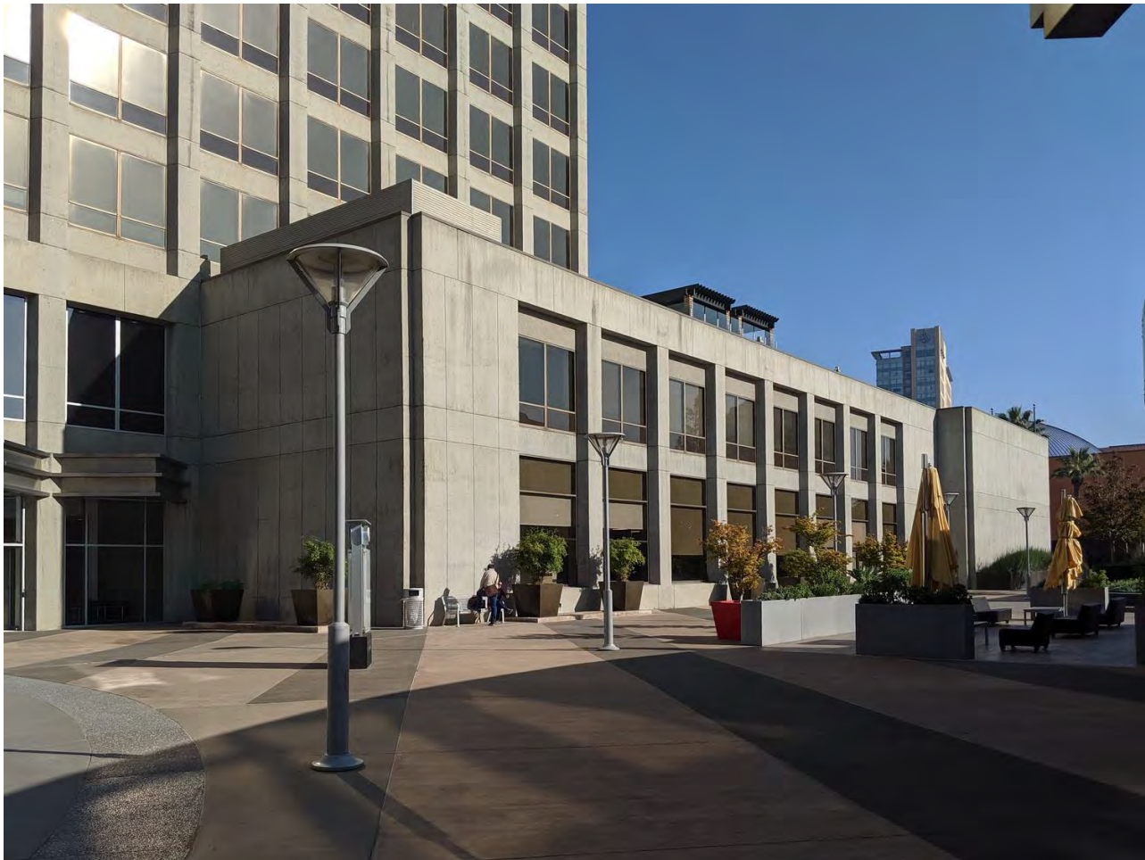
Two-story bank wing at plaza, viewed facing southeast.
