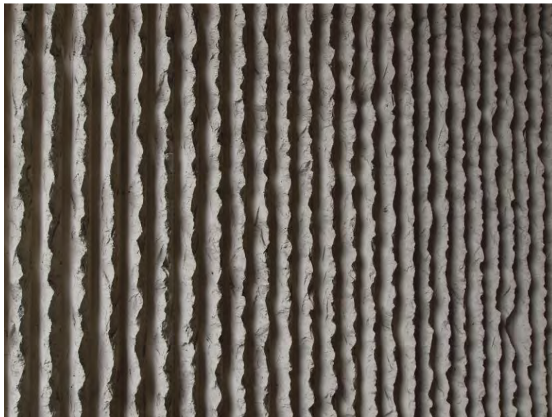
Board form concrete texture.
