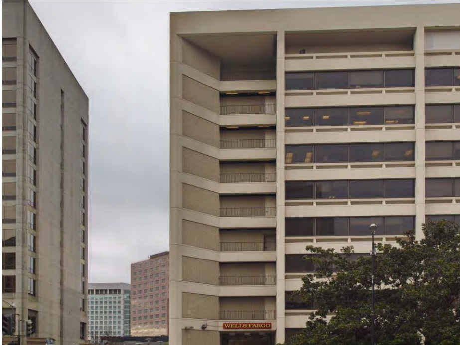
Upper façade (east) from across South Market Street.
