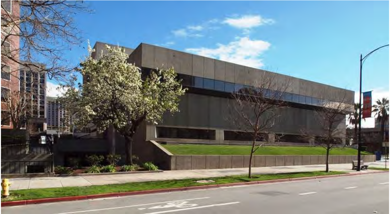
Almaden Boulevard façade, viewed facing southeast.
