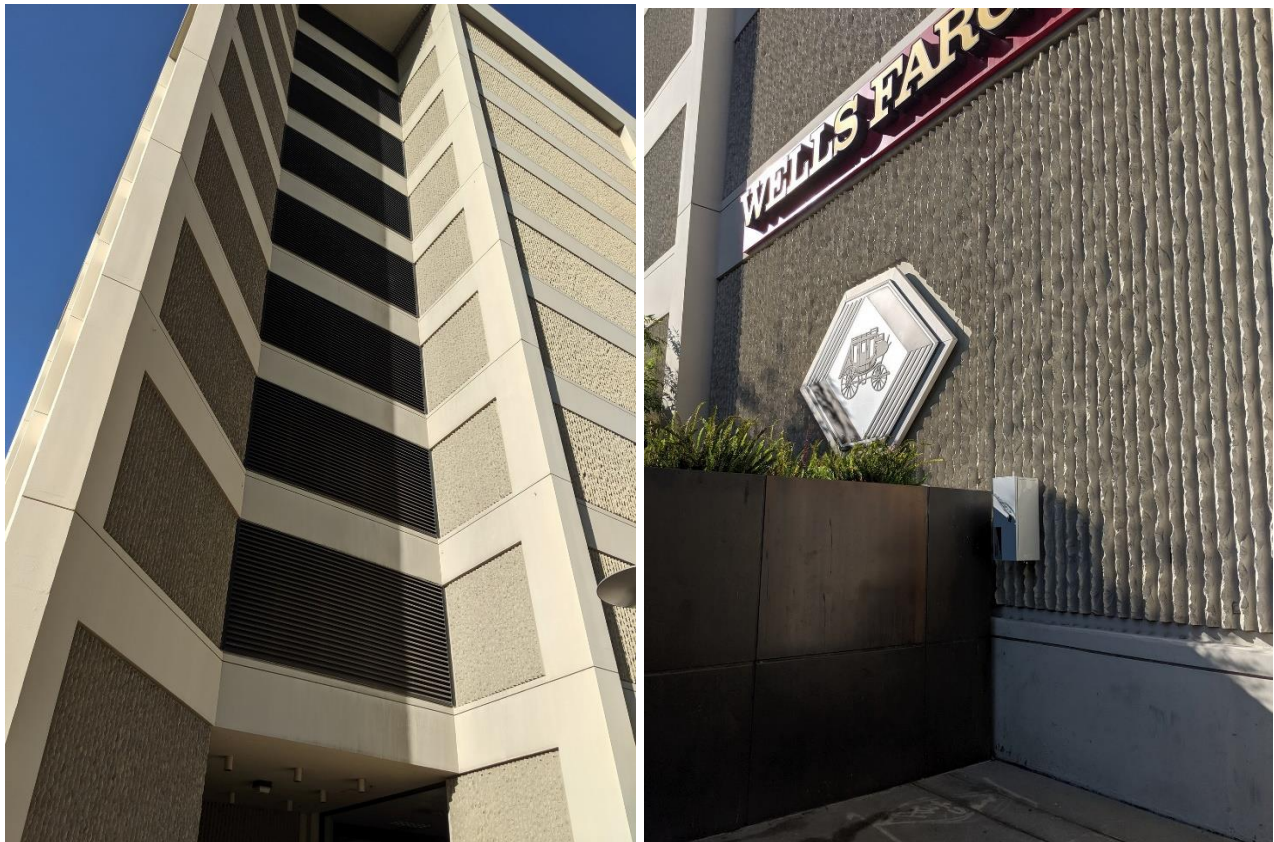
Brutalist detailing at south elevation of Wells Fargo Bank building at CityView Plaza showing vertically ribbed concrete panels.
