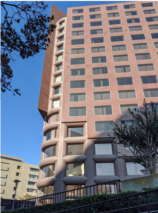
Front façade viewed facing north
