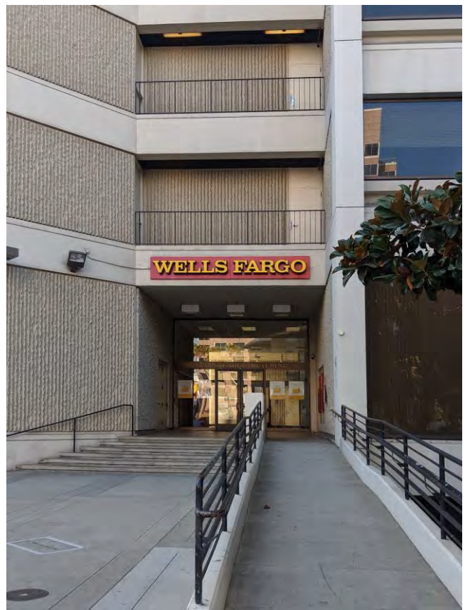
Building entry at South Market Street.
