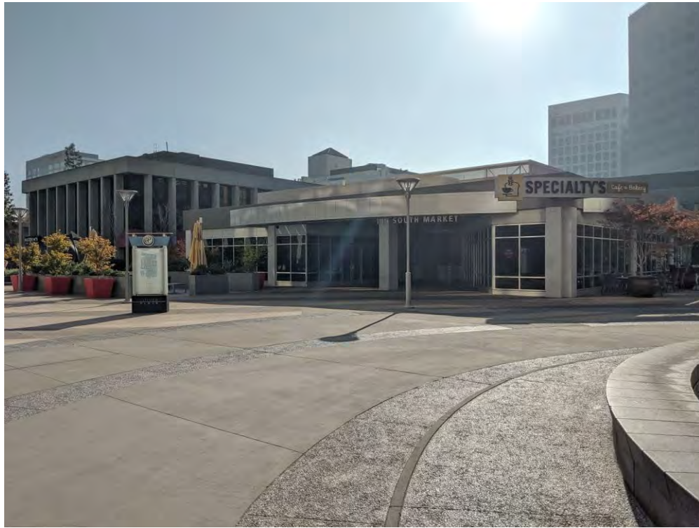
115 South Market St. pavilion and plaza deck, viewed facing southwest.
