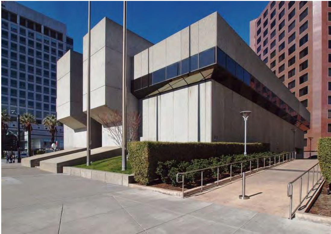
Park Avenue façade and east elevation, viewed facing northwest.
