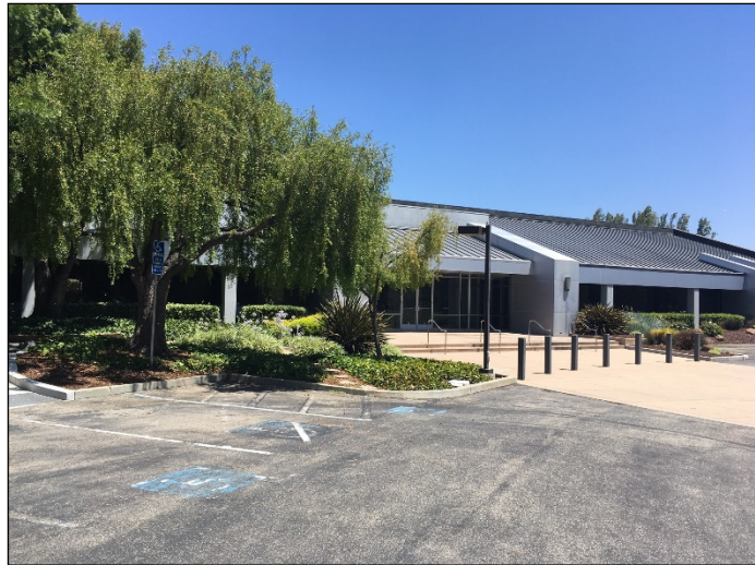
Photo 1. Developed/Landscaped Land Cover Type on the Project Site
