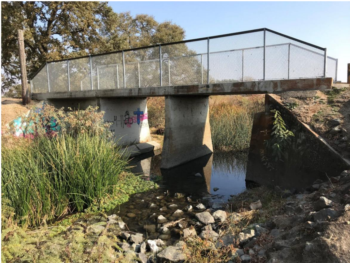
Photo 12: Looking Upstream at Bike Trail Bridge Downstream Face
