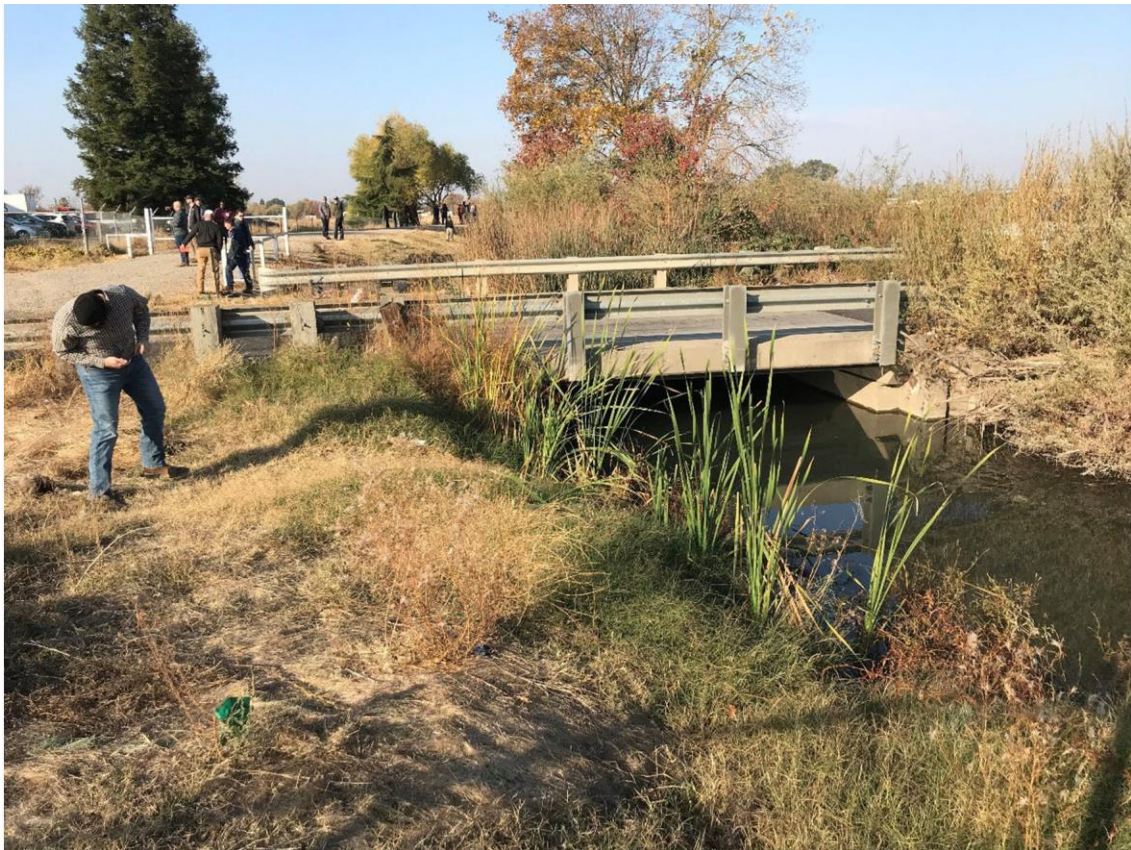
Photo 4: Bridge at Raley Blvd. Looking Downstream
