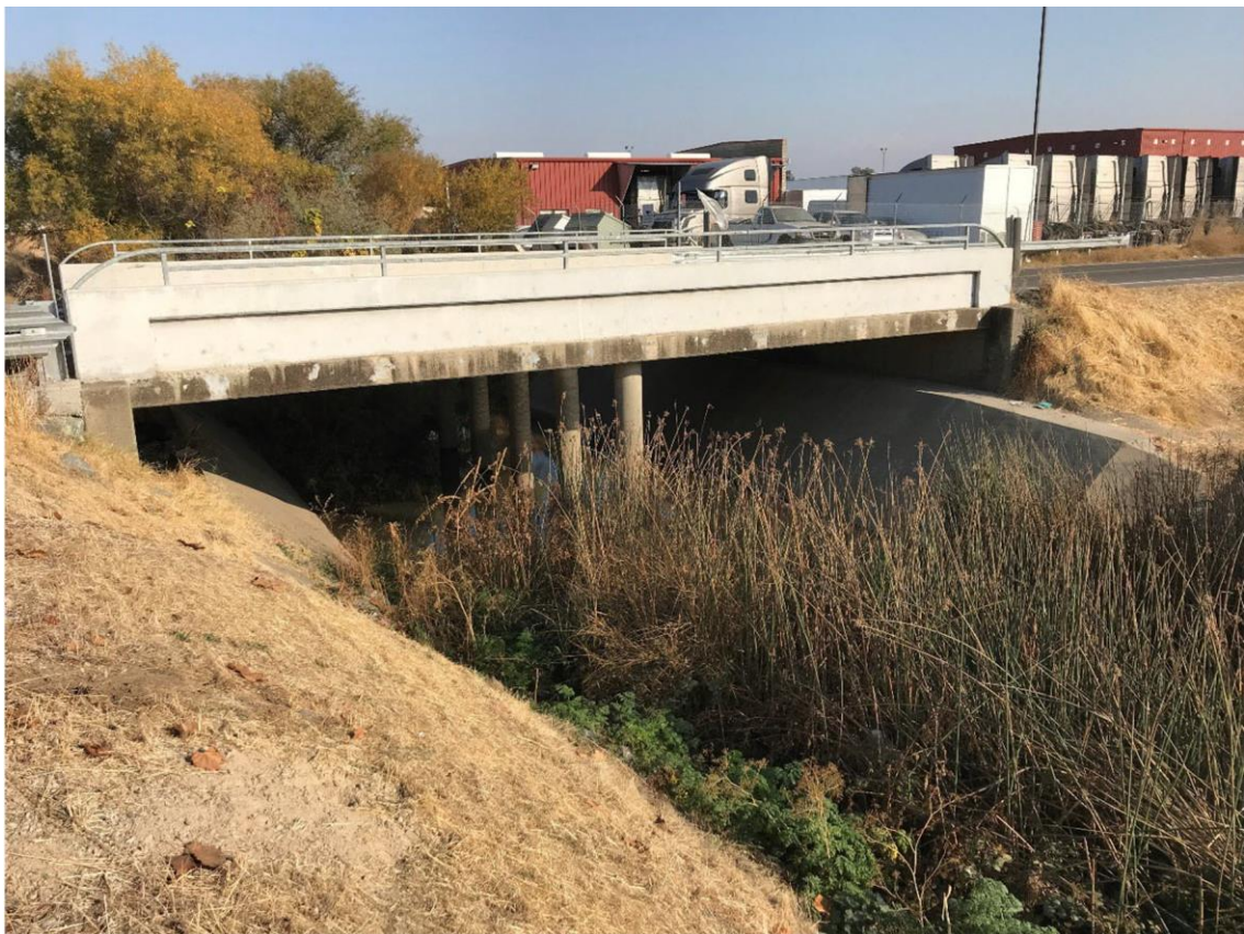
Photo 10: Looking Downstream at Vinci Ave. Bridge Upstream Face
