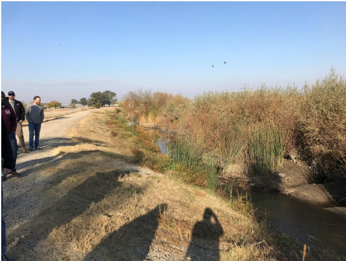
Photo 2: Looking Downstream from Left Descending Bank, Brush Noted
