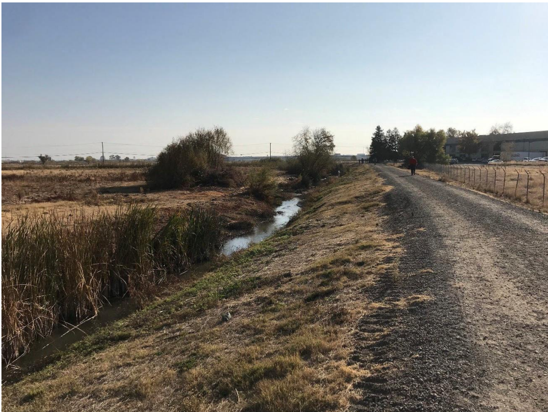
Photo 8: Looking Upstream from Left Descending Bank, (38° , 39' , 41.8" , -121° , 25' , 53.1")
