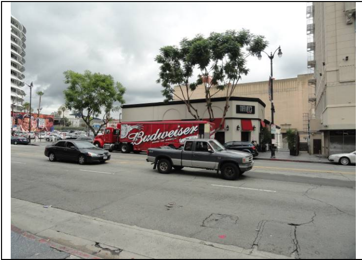
1. View of west side of subject property along North Vine Street, facing east.
