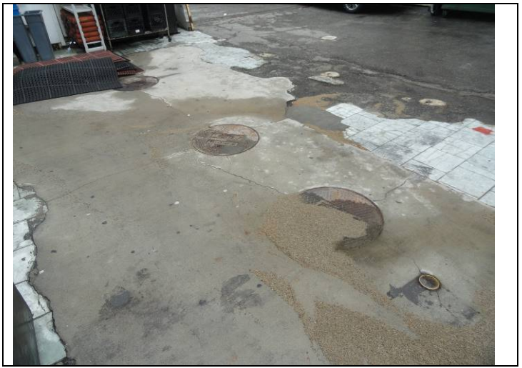
8. View of food grease interceptor on eastern portion of subject property.
