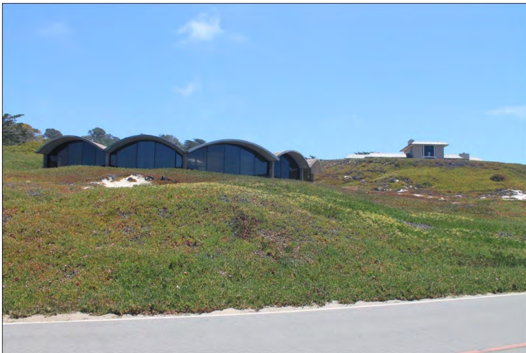
Figure 4.1-7. Several existing residences along 17-Mile Drive are seen extending above the ridgeline.
