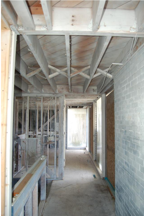
Photo 21 Demolished finishes in the upper level north wing.
