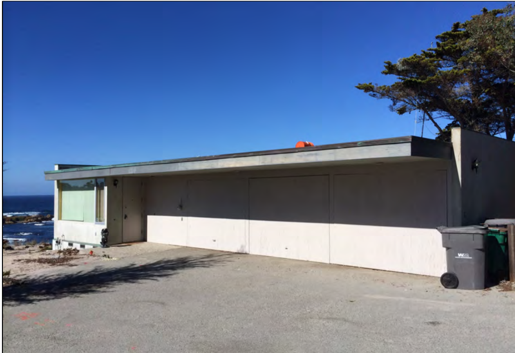
Figure 4.3-8. South elevation, looking northwest.
