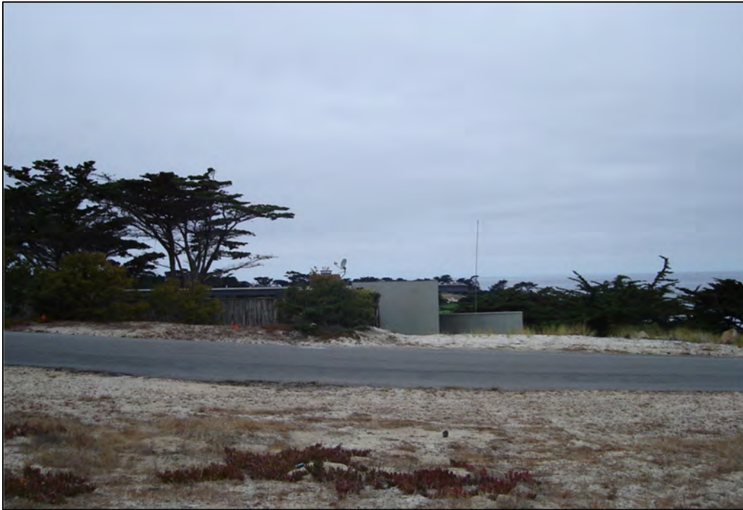
Figure 4.3-7. East elevation, looking west.
