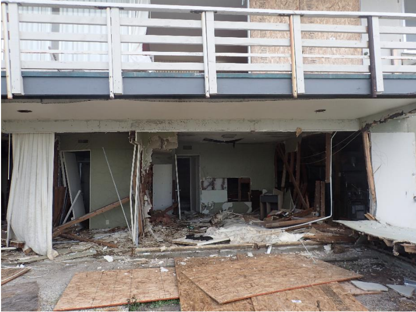
Photo 7 SWCA photo looking east from building's lower level, west side.
