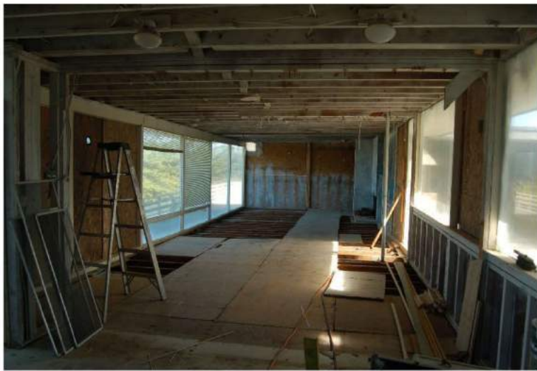
Interior of upper level has been gutted.
