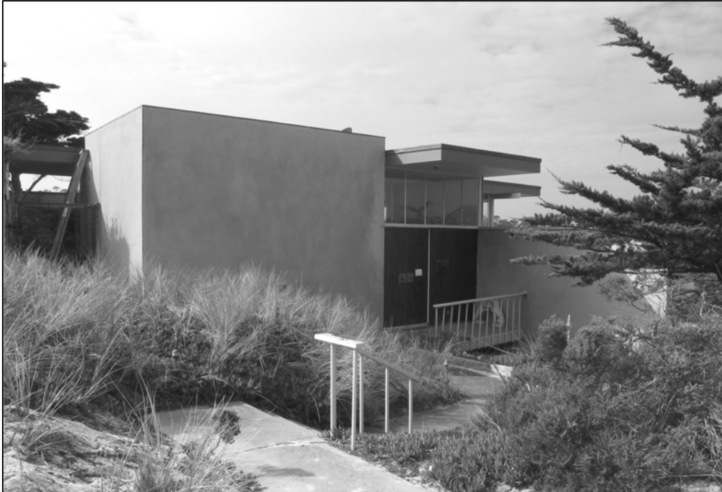
Figure 4.3-6. North elevation, looking southwest.
