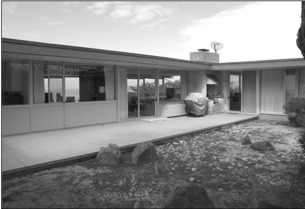
Figure 4.3-9. Looking northwest at east and north sides.
