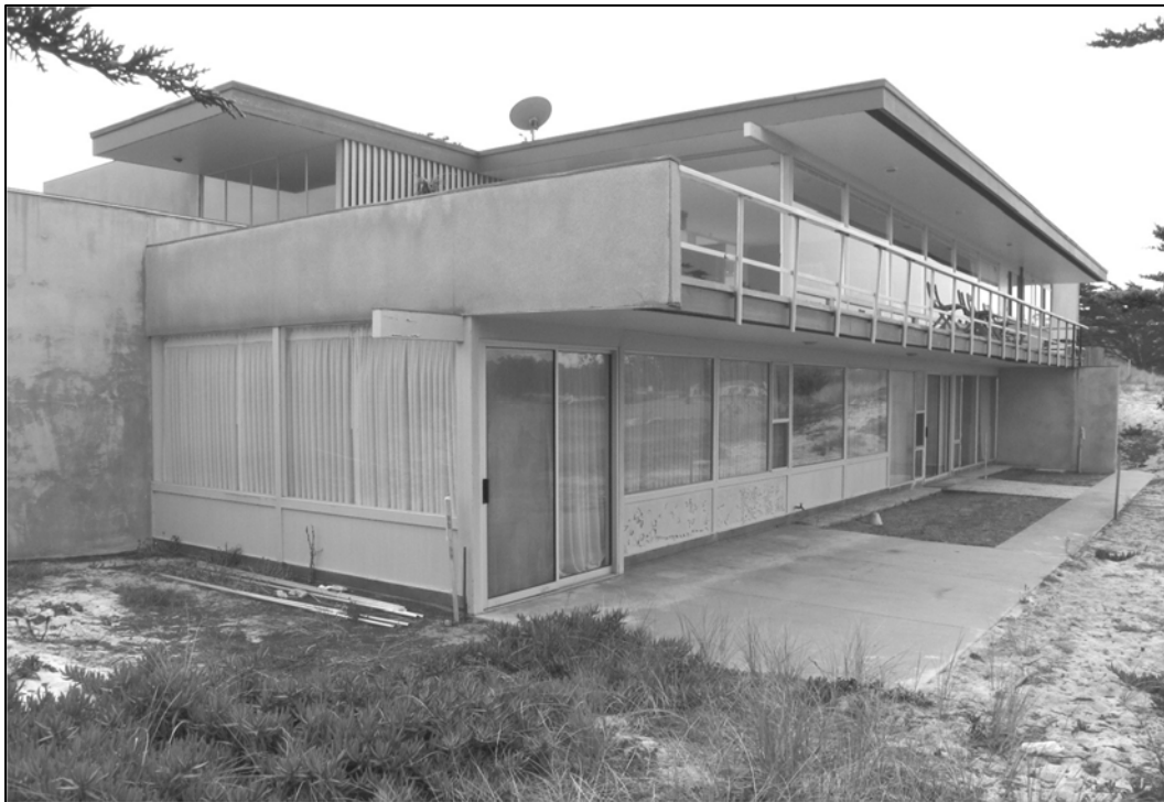
Figure 4.3-5. North and west elevations, looking southeast.
