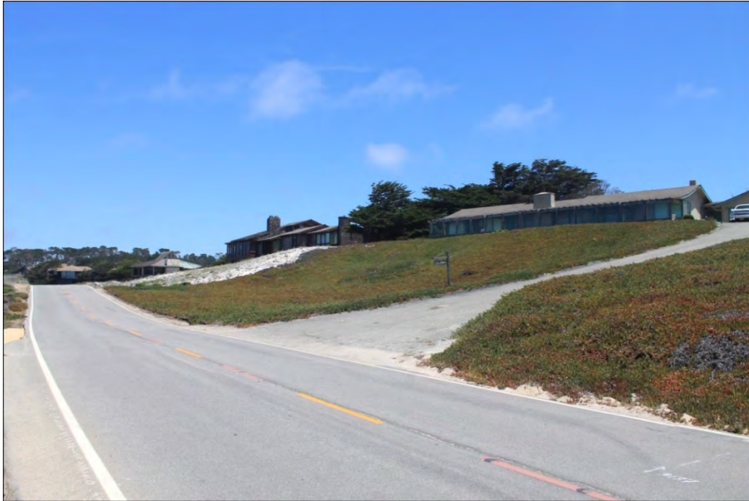
Figure 4.1-8. Existing residences along 17-Mile Drive.
