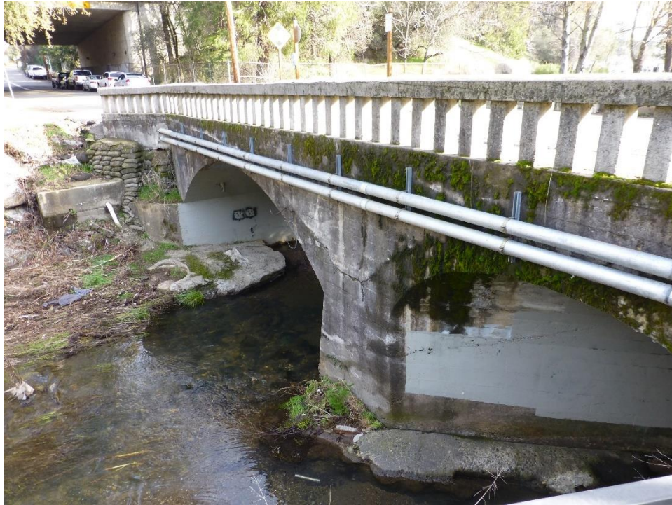
Photo 4.4-1 – Clay Street Bridge, Looking North
