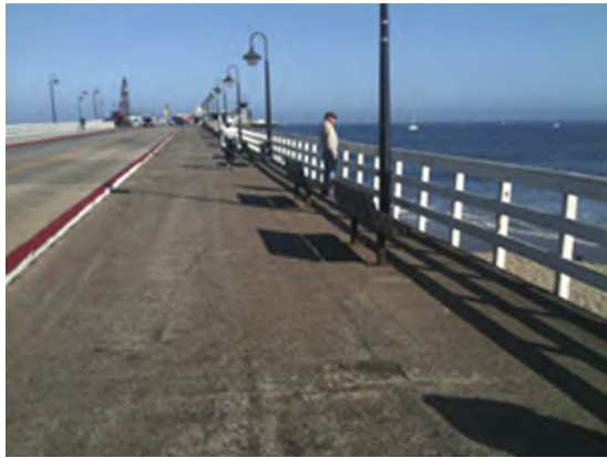
West Walkway Near Entrance
