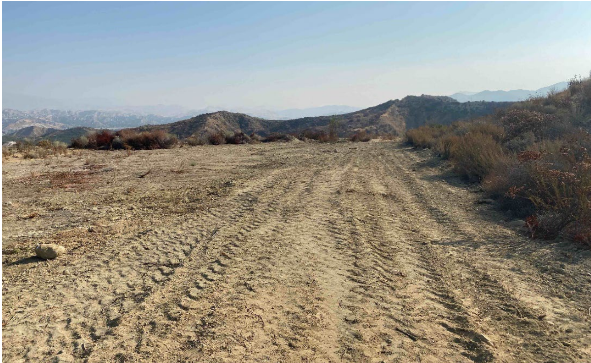
Photograph 1. View of Modified Project graded pad site, taken from southwestern portion of site facing northeast.
