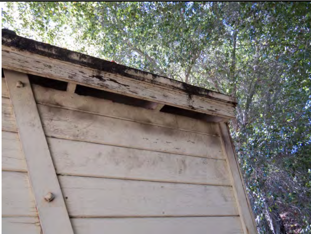
2. Eaves of structures were examined for bat entry and exit points. 3/21/2016
