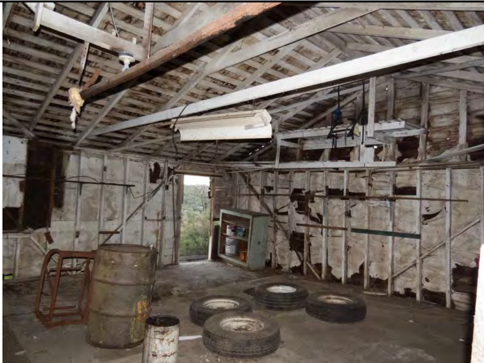
2. Interiors of structures were examined when access was available. 3/22/2016
