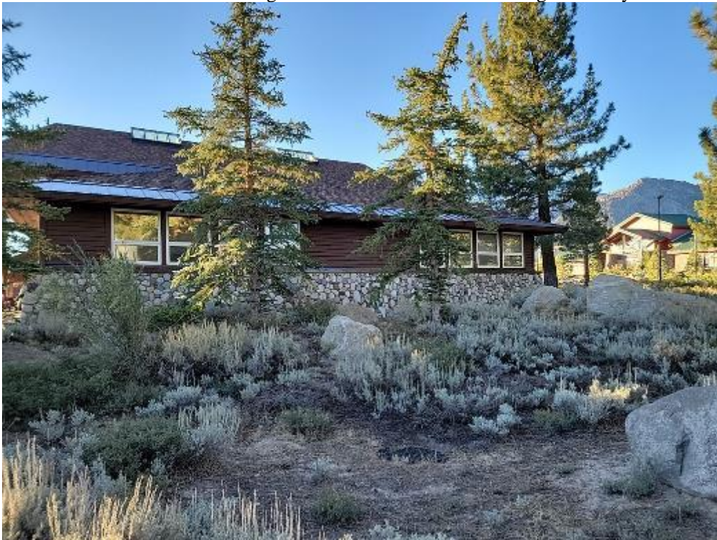
Photo 14. South-facing view from southwest corner of project site.
