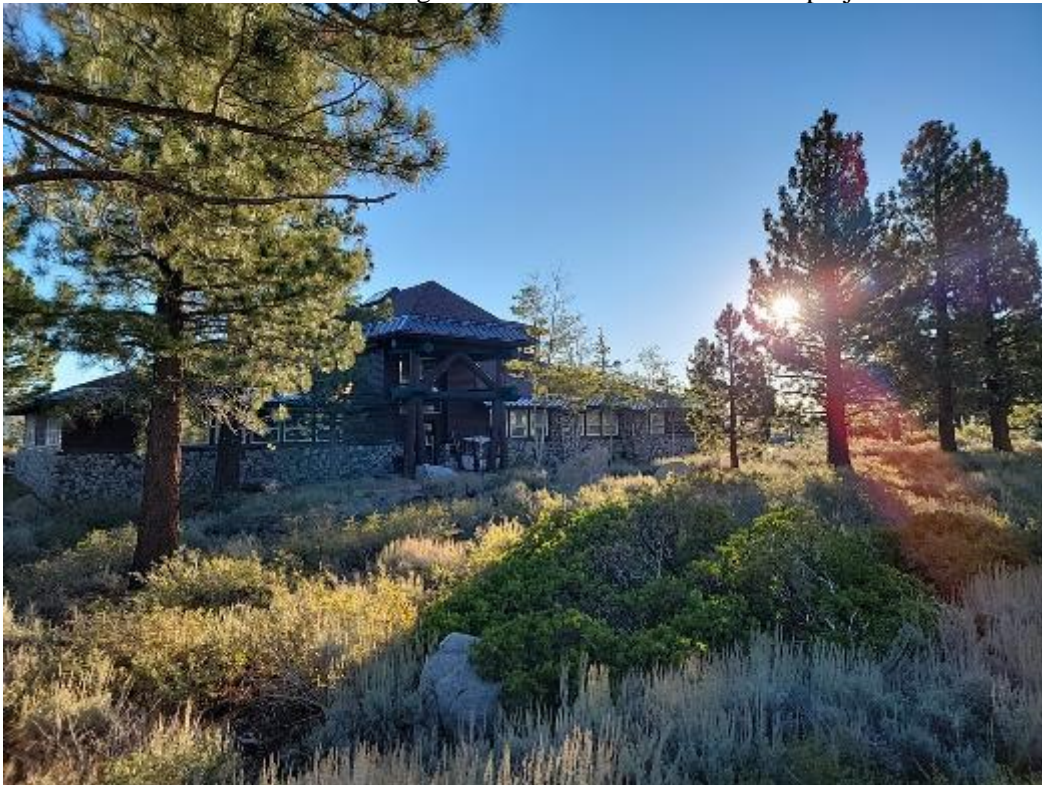
Photo 16. East-facing view from southwest corner of project site.
