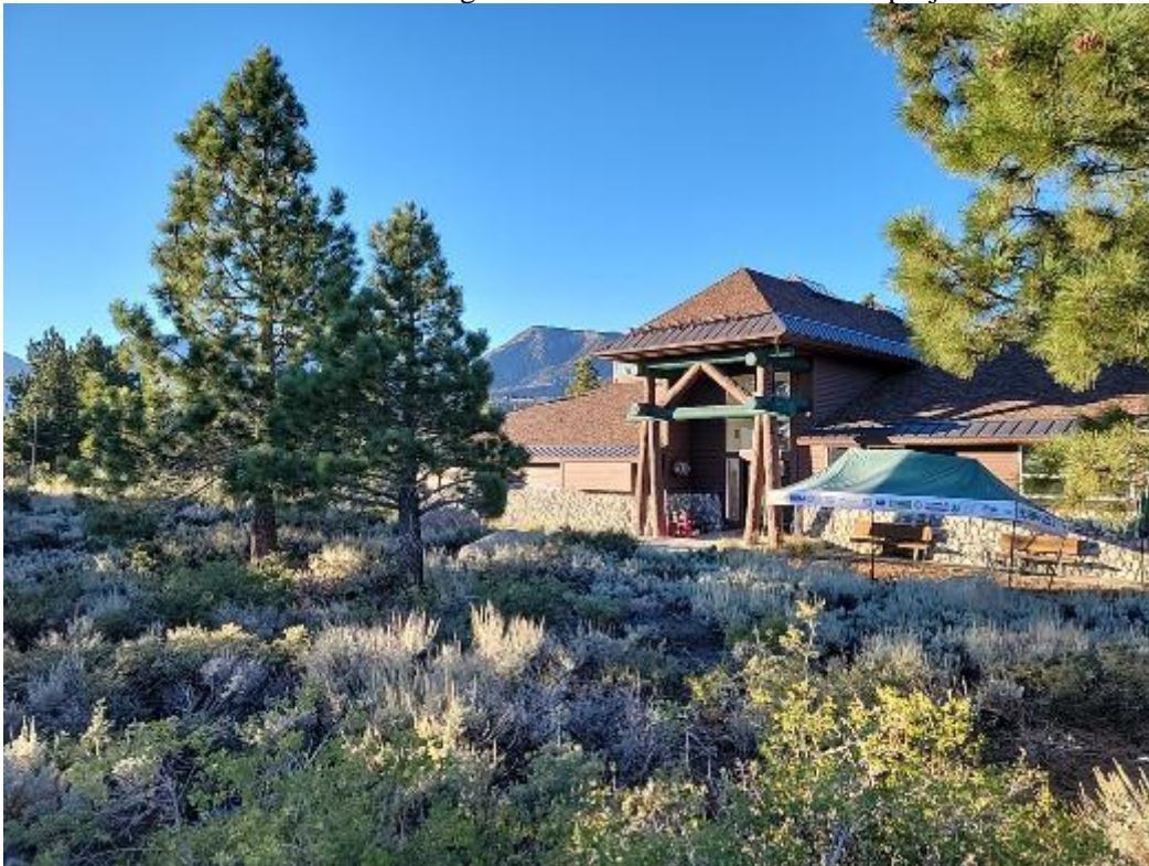
Photo 18. South-facing view from northwest corner of project site.
