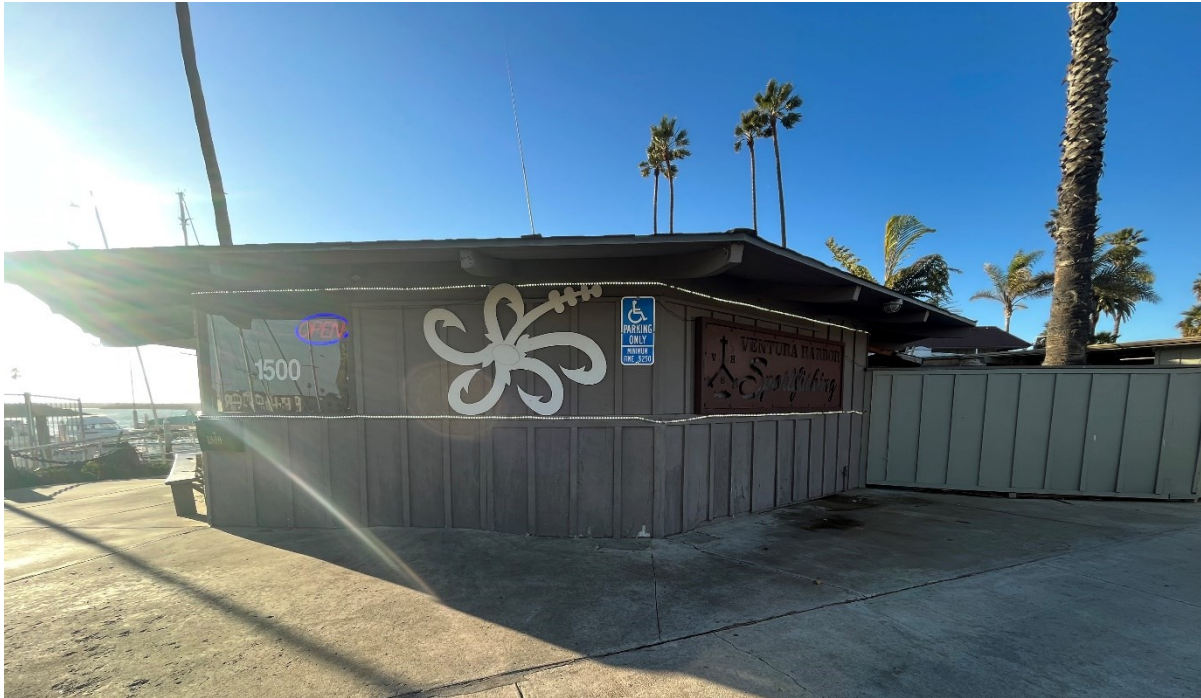
Figure 12 East Elevation of the Restaurant Building
