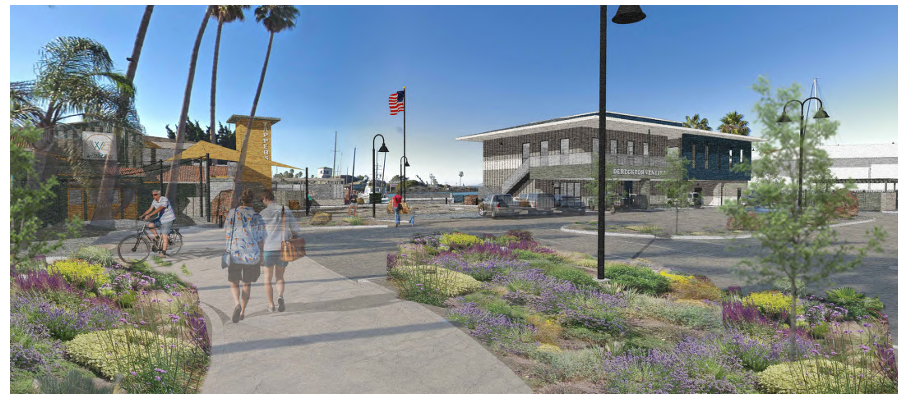
VIEW FROM ANCHOR WAY
