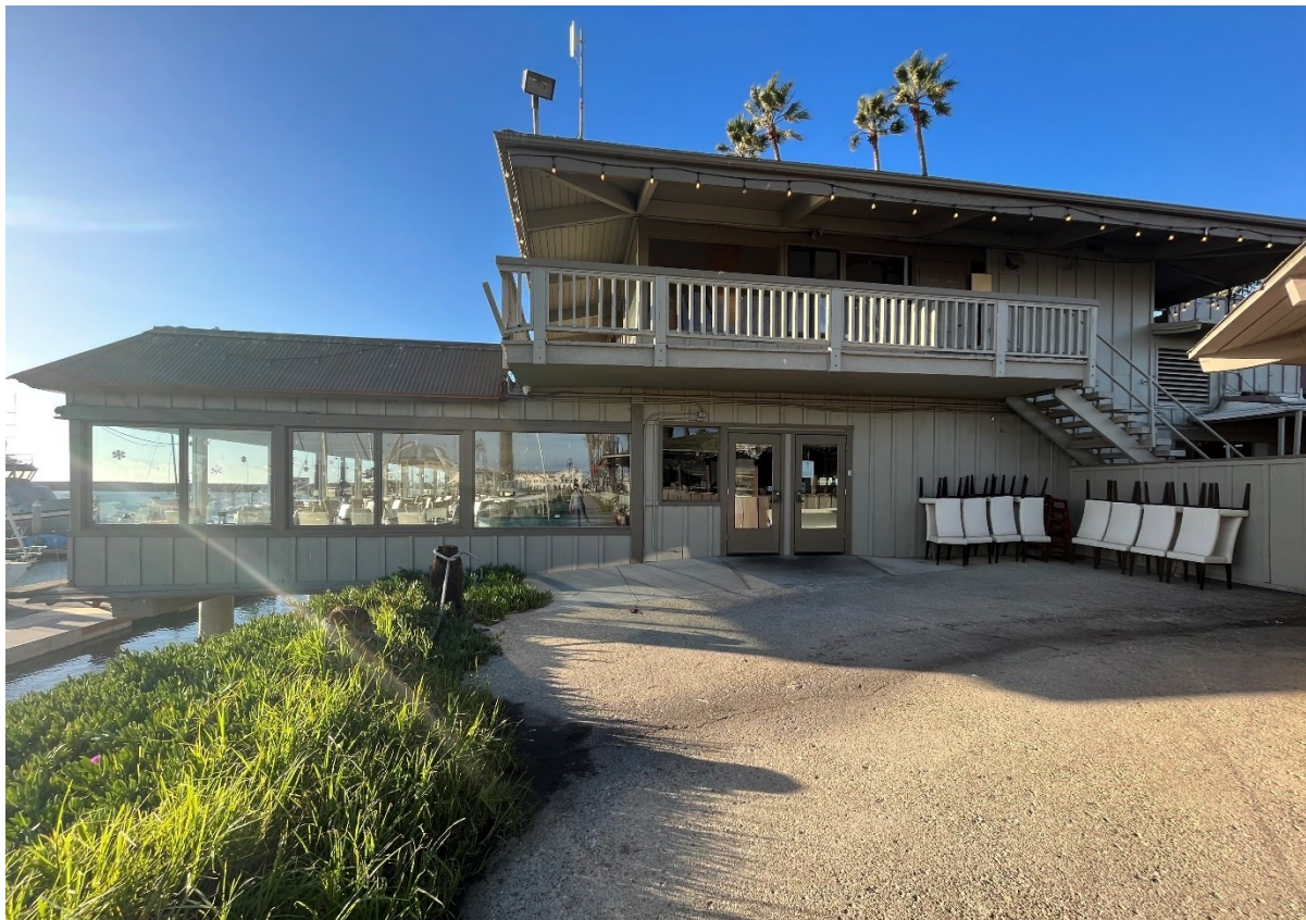
Figure 11 East Elevation of the Restaurant Building
