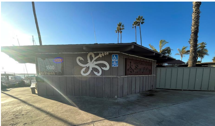
Photo 3: Sportfishing Building, View West
