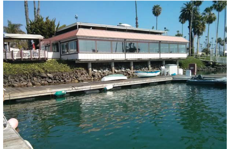
Photo 2: Existing restaurant on the project site.
