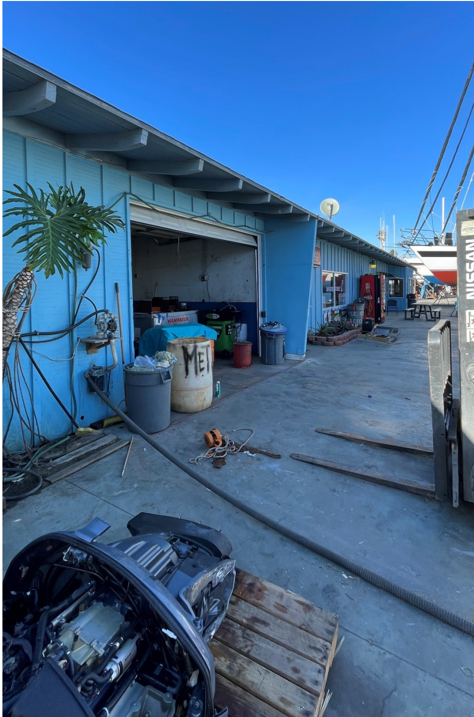
Figure 9 East Elevation of the Boat Repair Building
