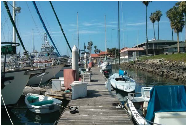
Photo 3: Existing dock structure and ramps to be removed.
