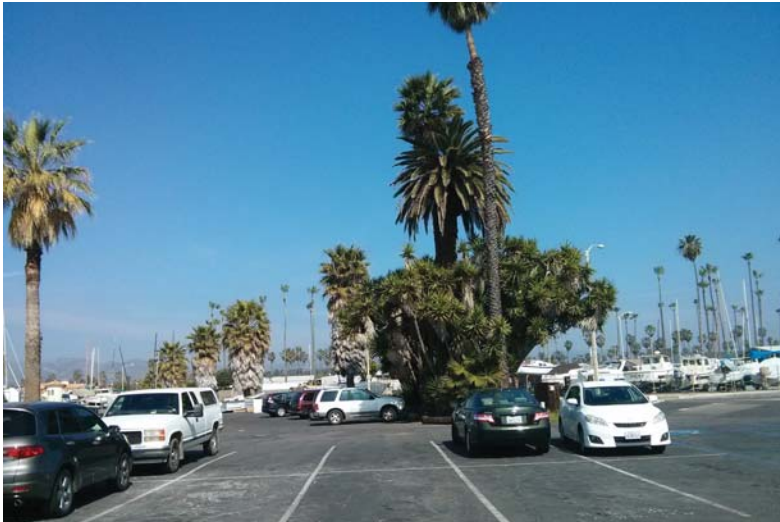
Photo 1: Existing parking lot to be repaved.
