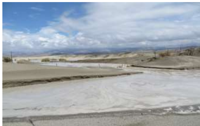
Photo 1: Flooding along Avenue 38, September 2014 Source: CVWD, 2014
