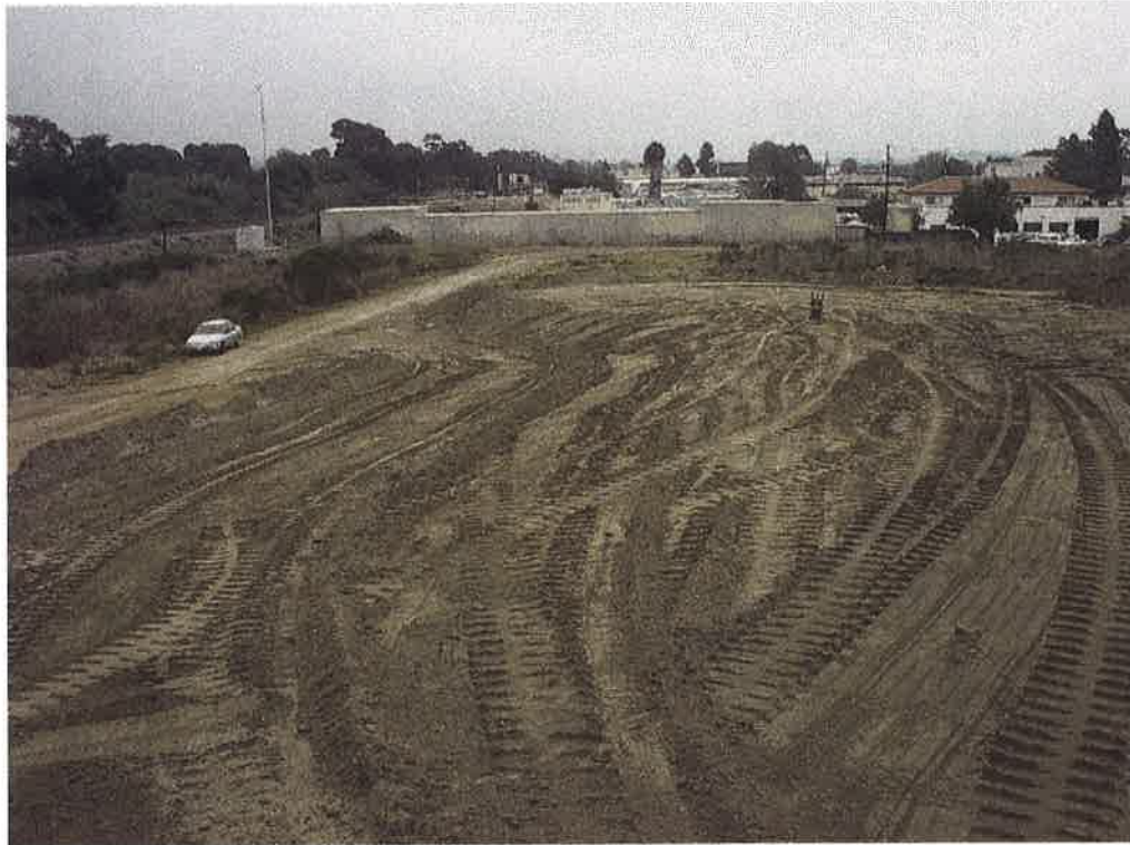
Looking east across stockpile after scraping to remove contaminated material.
