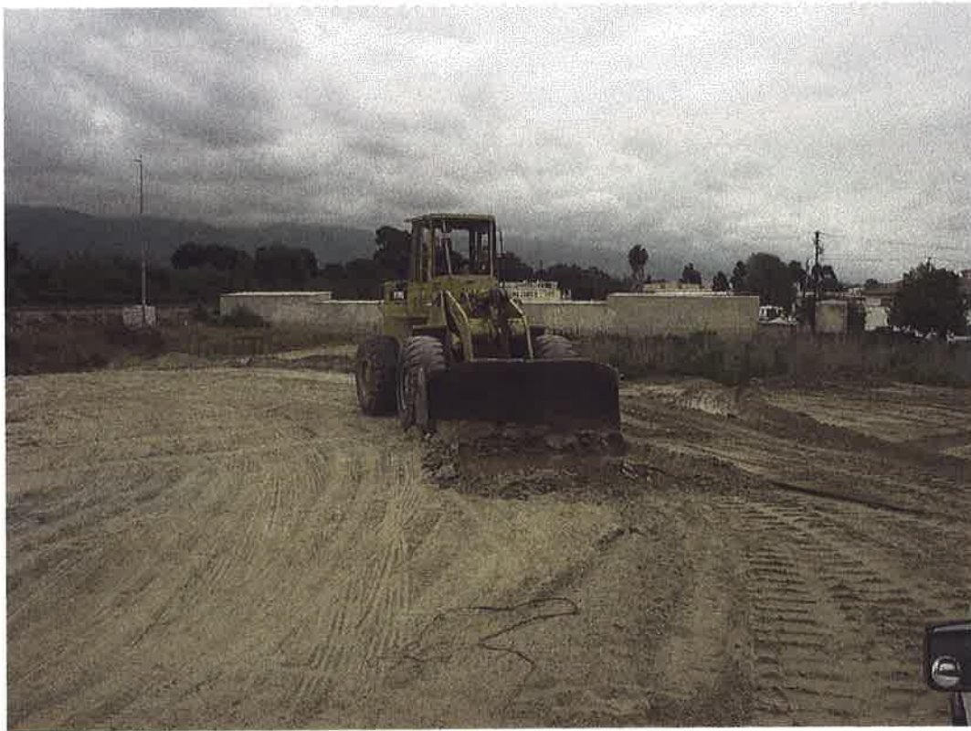
Removing contaminated material from localized areas after June 30 load-out
