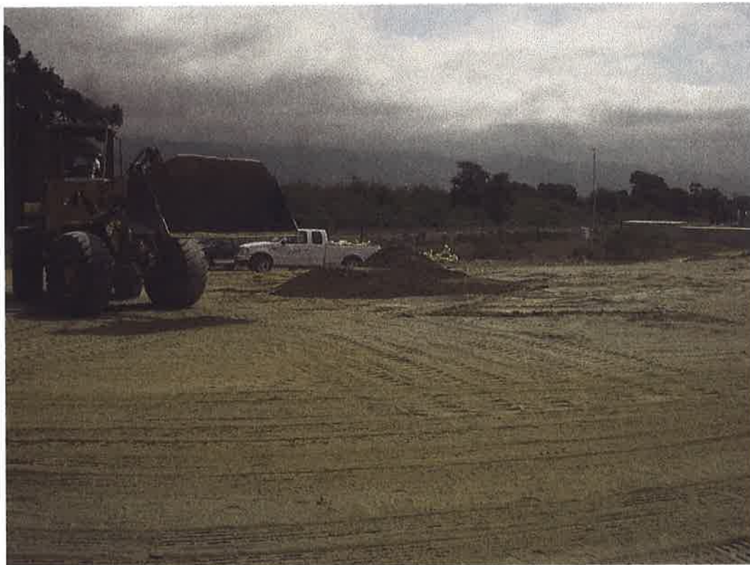
Final soil load-out to Santa Maria Landfill, July 1, 2004
