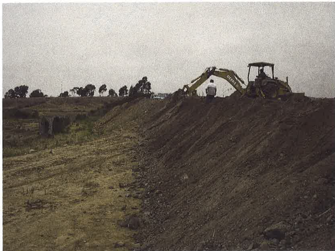
Backhoe removing contaminated material from slope face on south side of stockpile.
