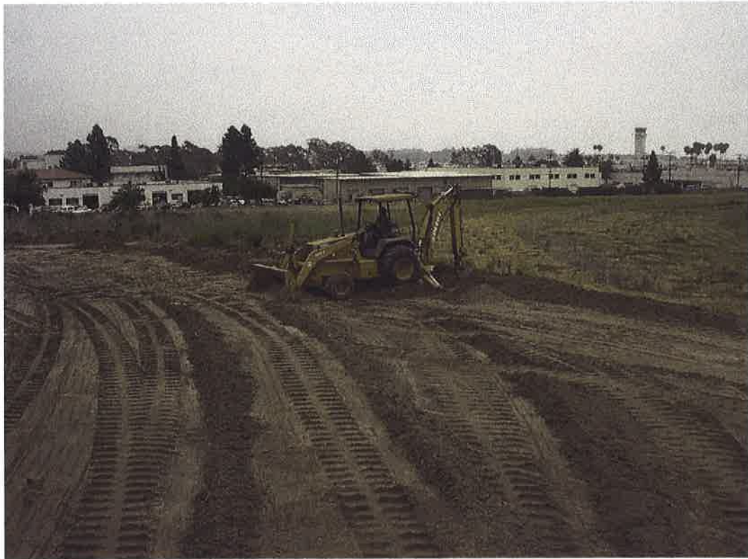
Backhoe removing contaminated material from slope face on south side of stockpile.
