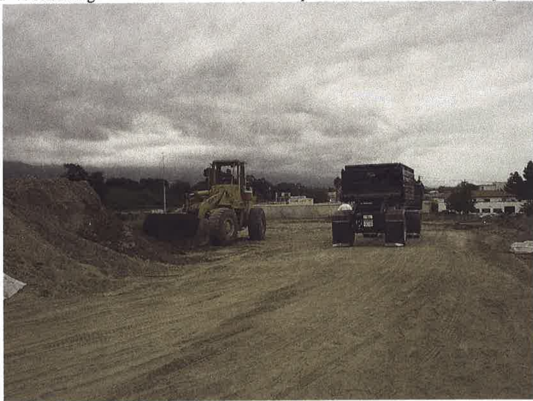
Initial soil load-out to Santa Maria Landfill, June 30, 2004
