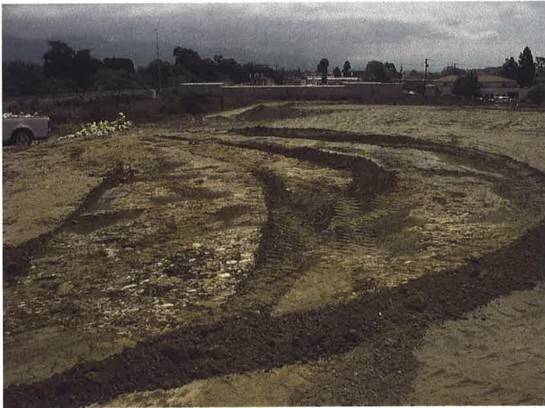
Stockpile area cleaned up after July 1, 2004 load-out
