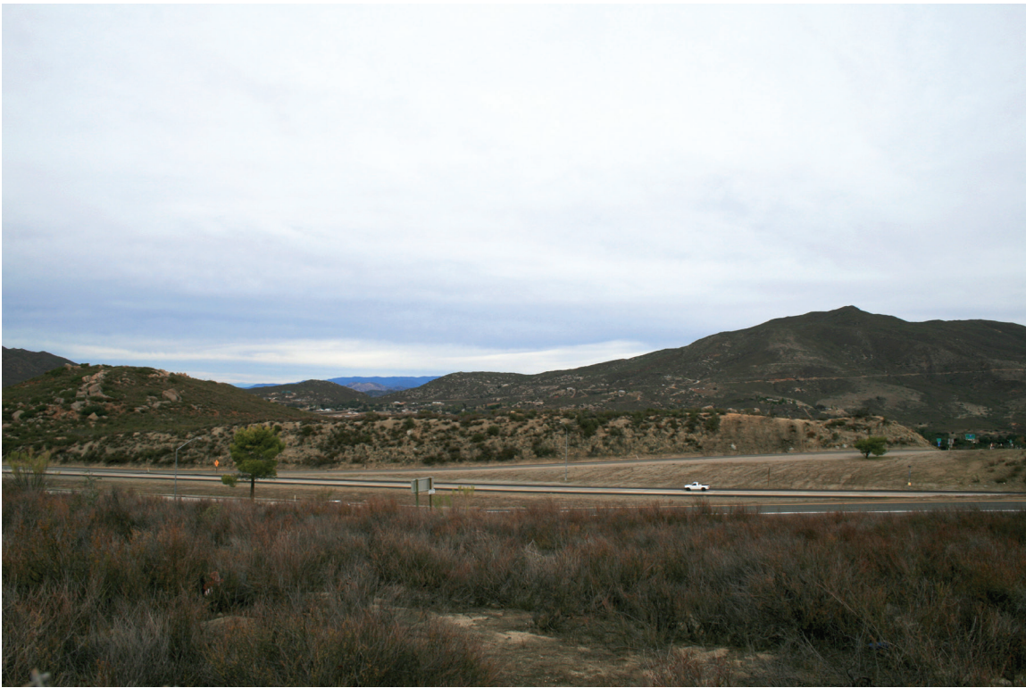
Near I-8 off-ramp, looking northwest
