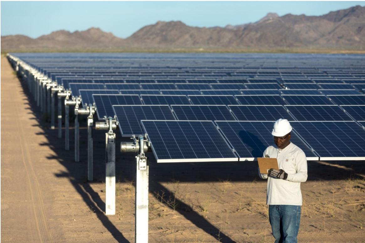
Figure A2. Typical Tracker Panel Configuration
