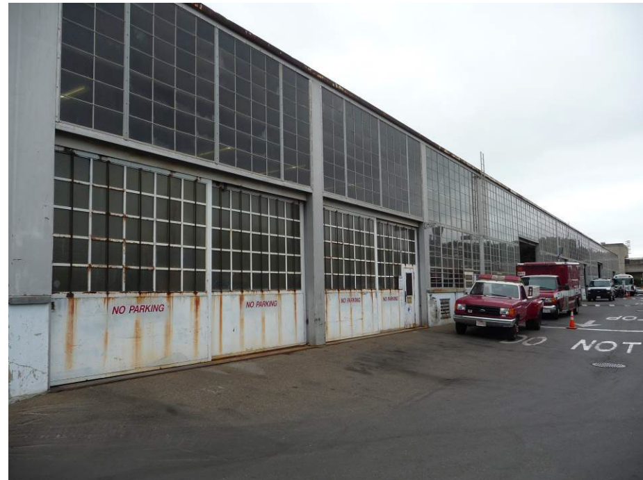
Building B facing northeast
