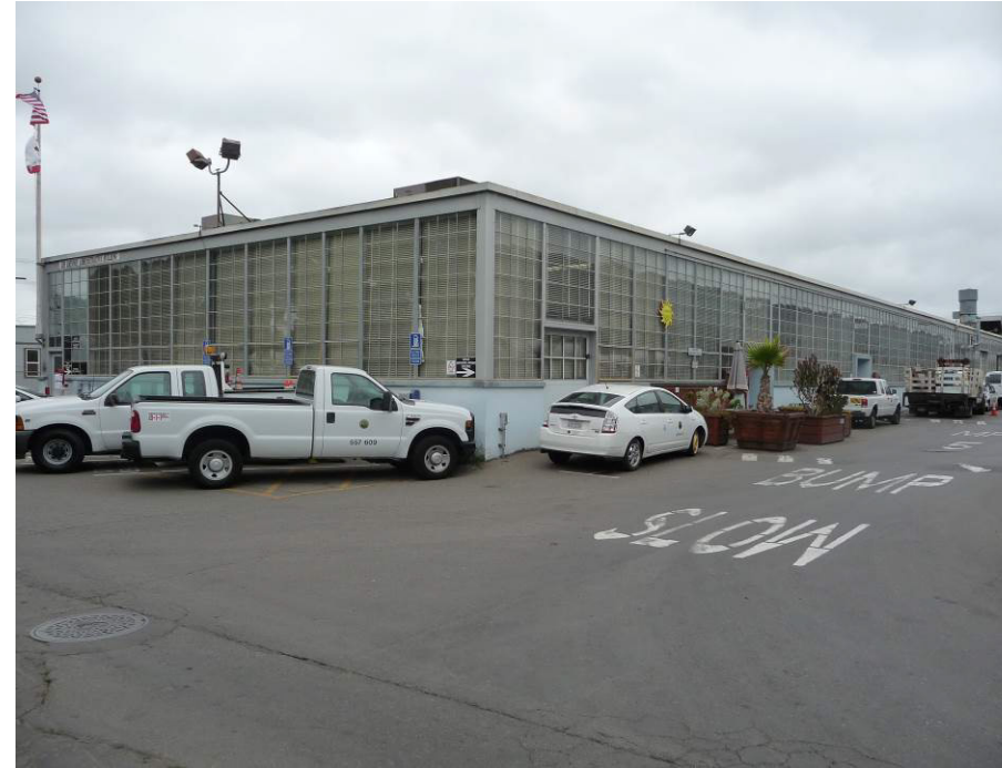
Building A facing west
