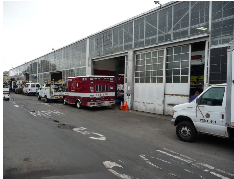
Building B facing southeast
