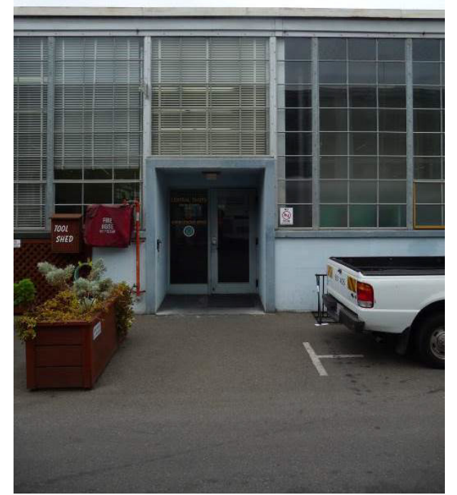
Building A facing southwest
