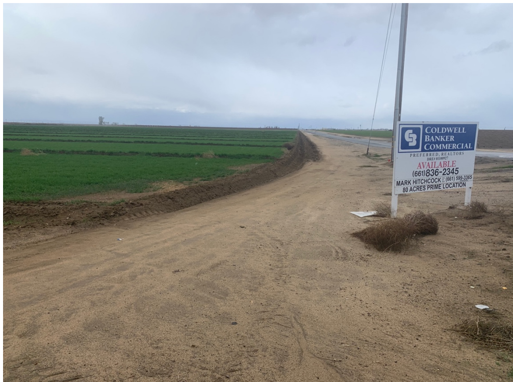
Figure A-4. Photograph of the project taken from the northeast corner of the project facing southwest (25JAN21).
