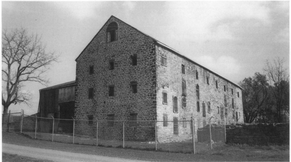
Figure 24. Once mothballed, a property must still be monitored and maintained. The openings in this historic barn has been modified with a combination of wood louvers and metal mesh panels which require little maintenance. The grounds are regularly mowed, even inside the chain link security fence. Photo: Williamsport Preservation Training Center, NPS.
