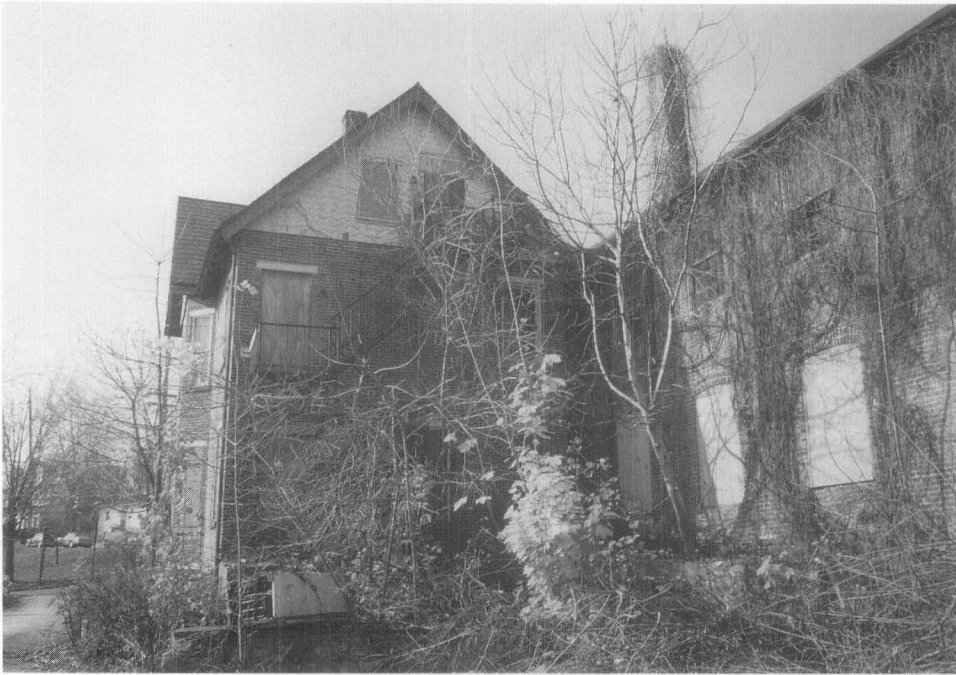
Figure 2. Improper treatment: Boarding up without adequate ventilation, lack of maintenance, and neglect of this property have accelerated deterioration. Photo; NPS file.
