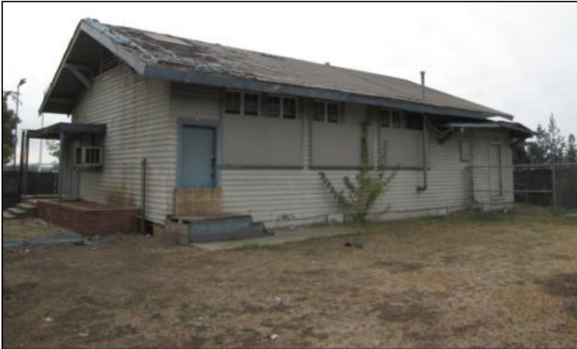
The Old Schoolhouse building, front and north elevation. View facing southwest.
