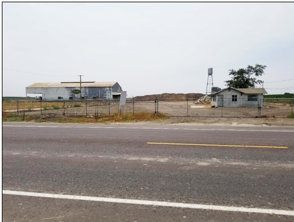
Figure 3. Standing structures within batch plant project area, looking south from Avenue 280.
