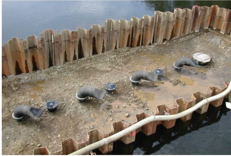
Figure 2-11. Examples of Duckbill Valves to be Use on Ocean Outfall
