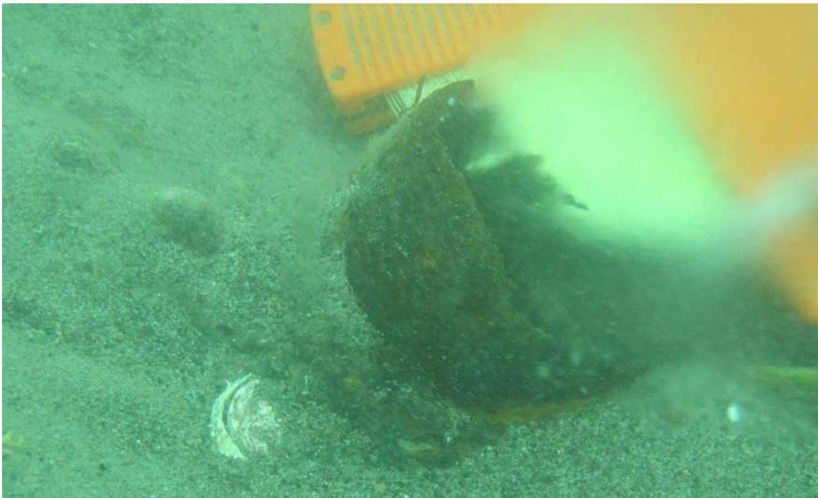
**Photograph 16.** Broken ocean outfall diffuser. Note diffuser actively discharging low saline water.
