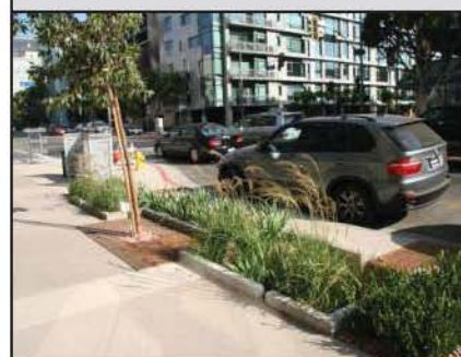
Bioretention Source: Geosyntec Consultants
