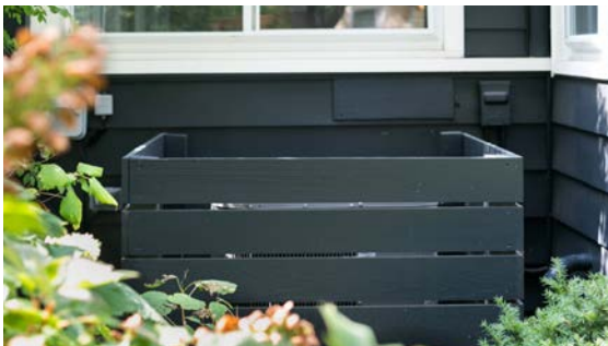
Photo 7.16 - Example of mechanical equipment screen
