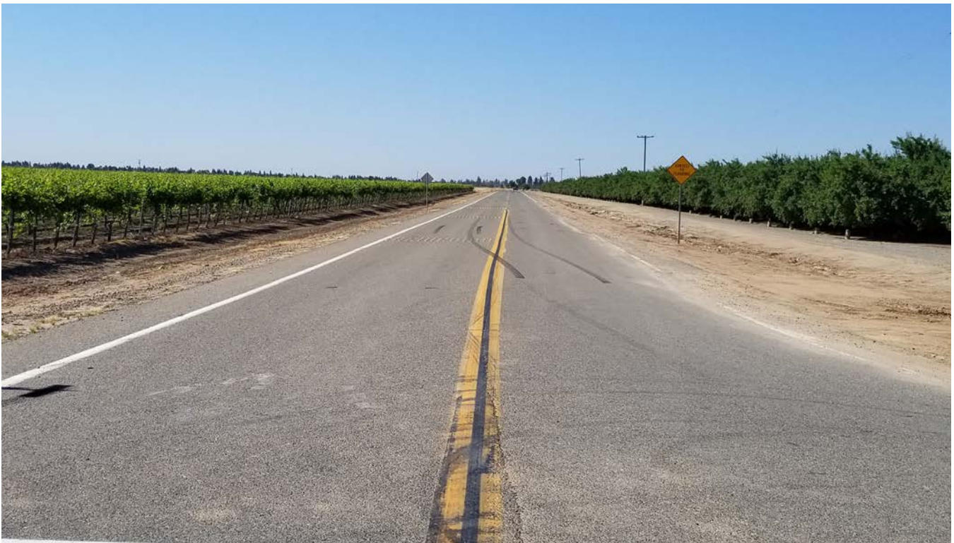
Photo 3.1 - Looking South at the intersection of Road 24 and Avenue 16
