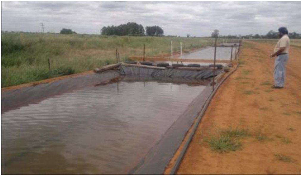
Figure 20: Lined sections of an old irrigation channel at Yanco Agricultural Institute. (Photograph: A. Leung)
