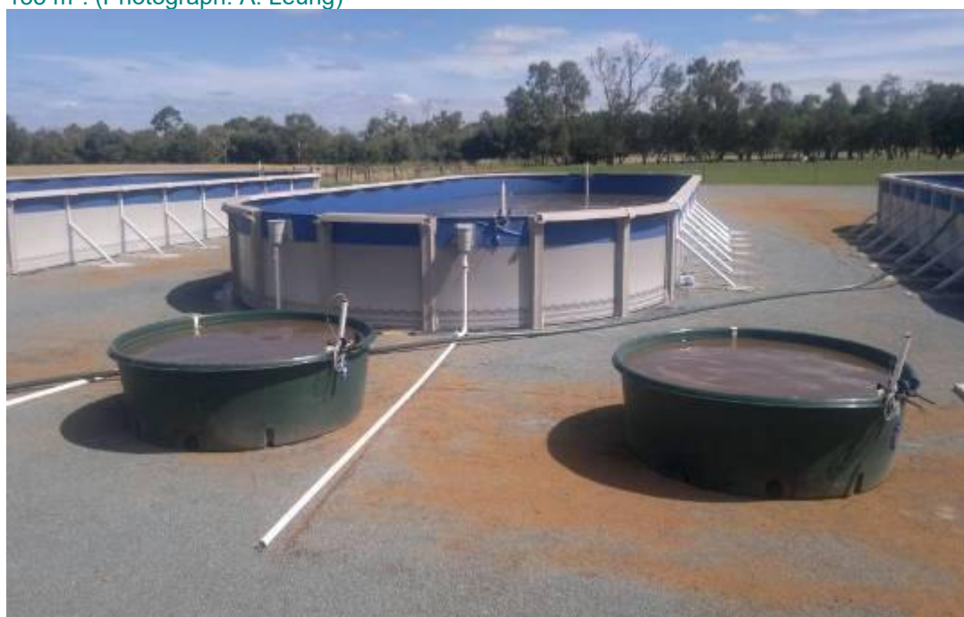
Figure 19: Large evaporation ponds installed at Dookie. Each pond has a surface area of 135 m 2 . (Photograph: A. Leung)
