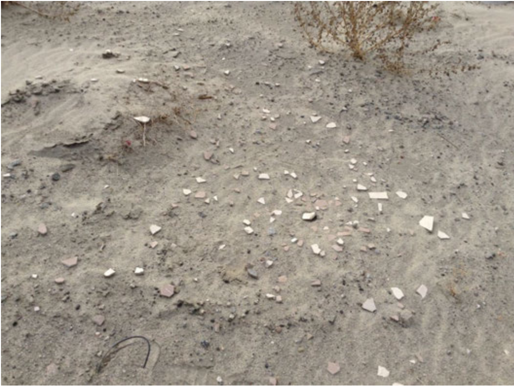
Photo 19: Scattered debris on the south edge of the Property (broken floor tile)
