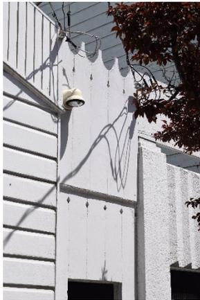
Figure 7. Decorative sawn roofline pattern at the wood wall enclosing the pedestrian alley at 63 Brady Street.
