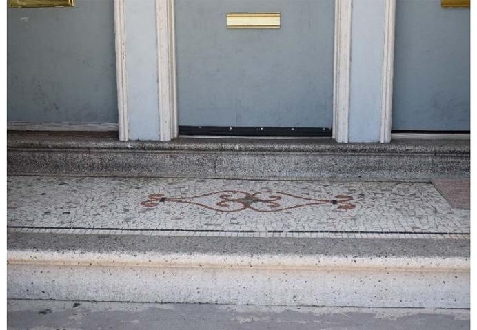
Figure 2. Detail of the mosaic tile on the floor of entry vestibule.
