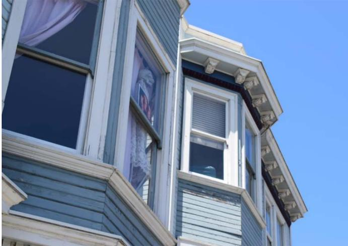
Figure 1. Detail of the narrow channel siding and wood double-hung windows at the primary façade.
