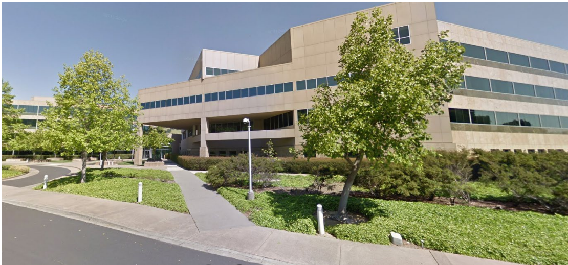
Graphic 1. Four-story office buildings at former Fireman’s Fund campus (source: Google Maps, 2023)
