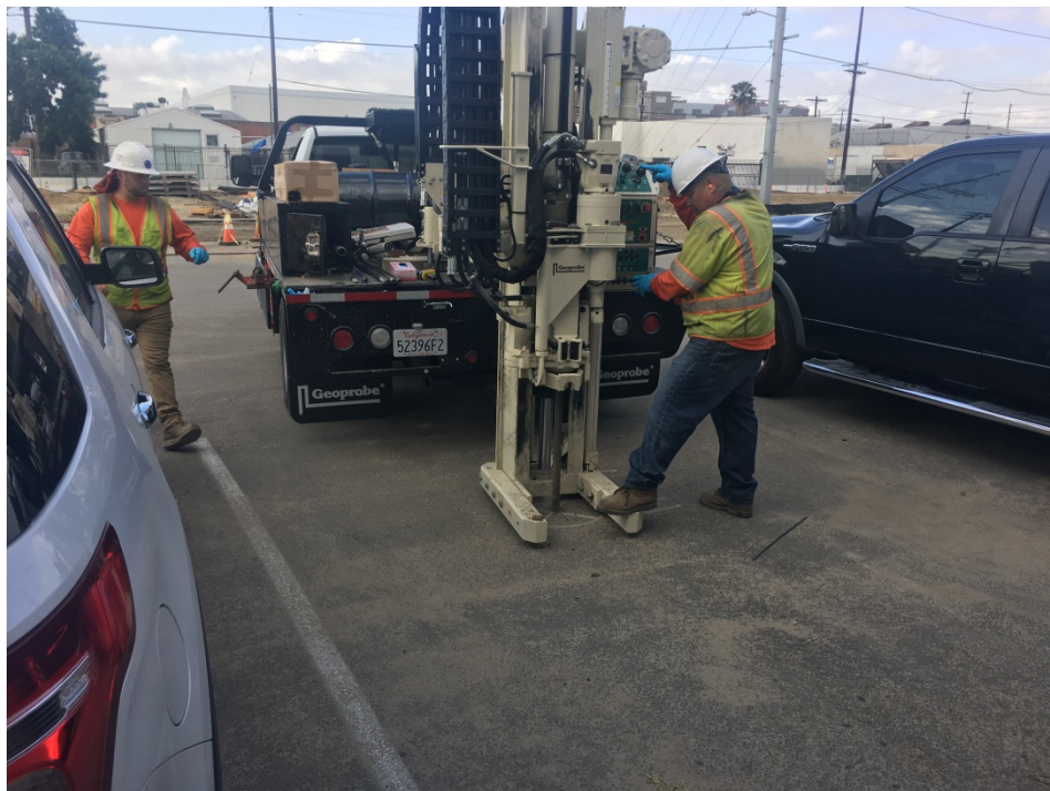
b. Direct Push Drill Rig Penetrating the Asphalt Layer at Soil Boring 1A-4
