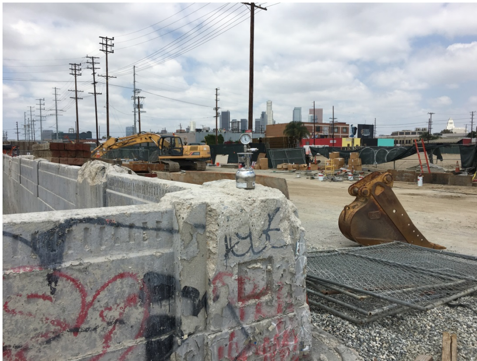
b. Obtaining Ambient Air sample in Area 2A using Summa Canister
