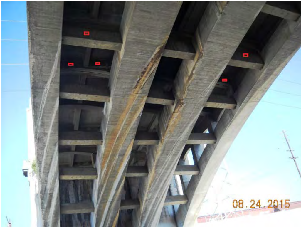
Photo 9: Approximate locations selected for placement of alternative bat habitat enclosures on the concrete girders of the Fourth Street Viaduct; view facing east
