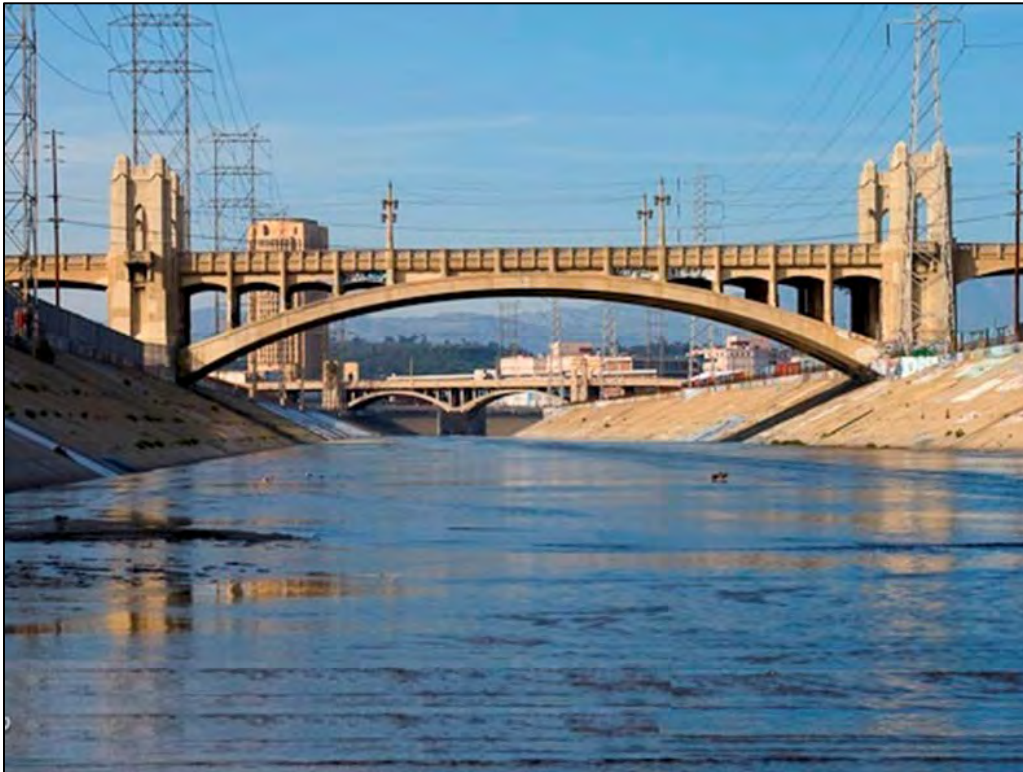
Photo 1: Fourth Street Viaduct over the Los Angeles River; view facing north
