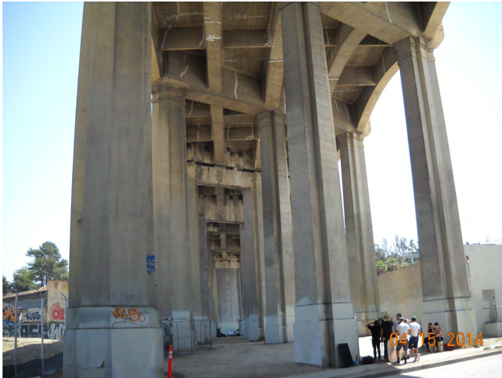
Photo 1: Solid concrete piers and girder structure on viaduct; view facing east
