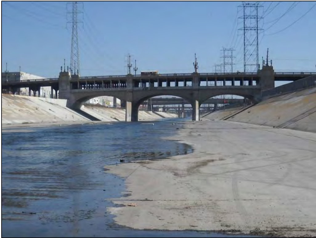
Photo 5: Seventh Street Viaduct over the Los Angeles River; view facing south
