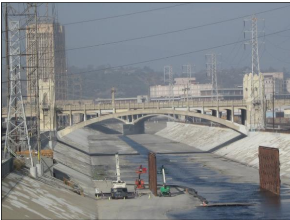
Figure 4: Fourth Street Viaduct (LAHCM #904 and Bridge No. 53C0044) (GPA, 2017)
