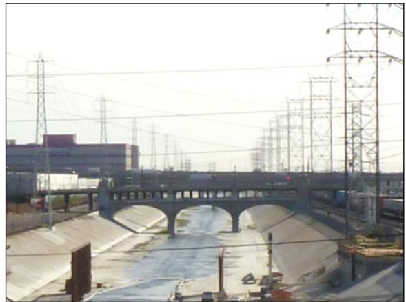
Figure 5: Seventh Street Viaduct (LAHCM #906 and Bridge No. 53C1321) (GPA, 2017)
