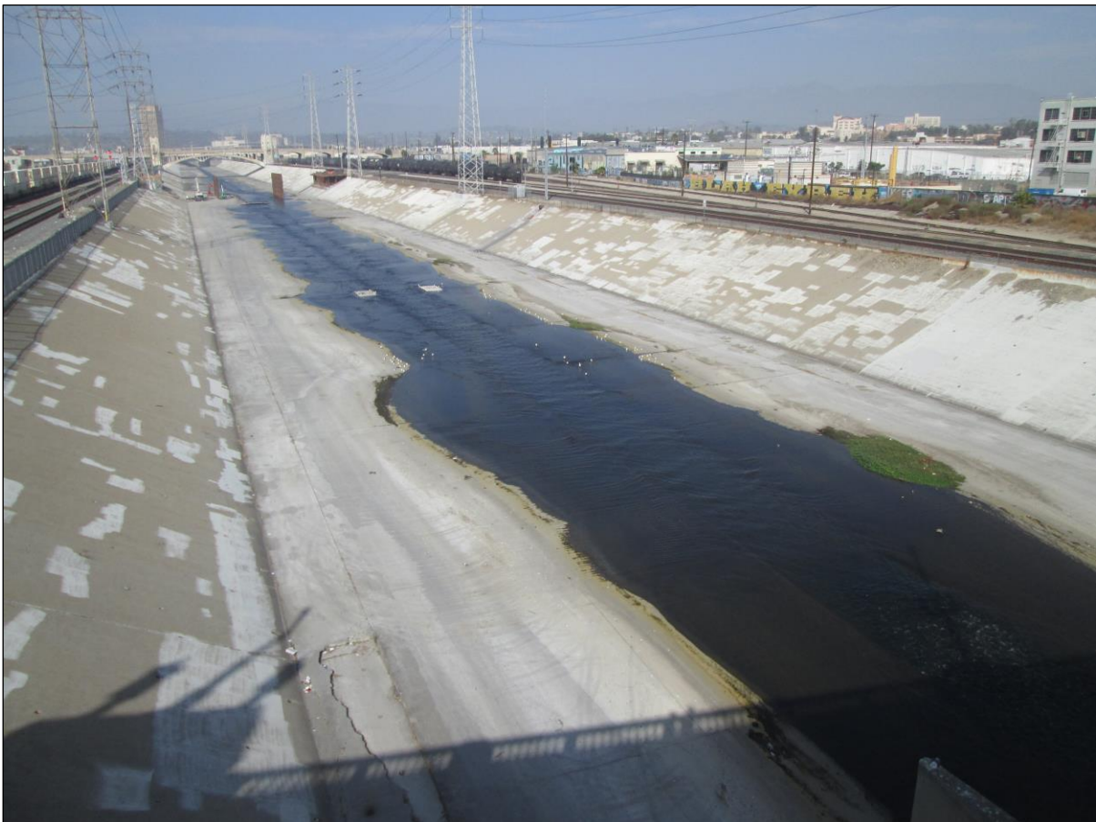
Figure 6: Los Angeles River, segment within the Project Study Area, view facing north from Seventh Street Viaduct (GPA, 2017)
