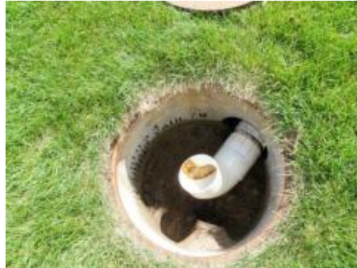
Figure- Concrete outlet vault with adjustable "swing joint" to control water elevation.
