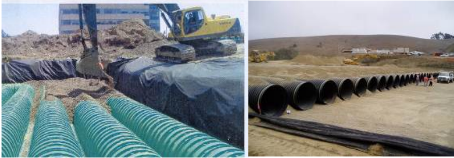
Figure- Triton S-29 Chambers with EPDM liner
