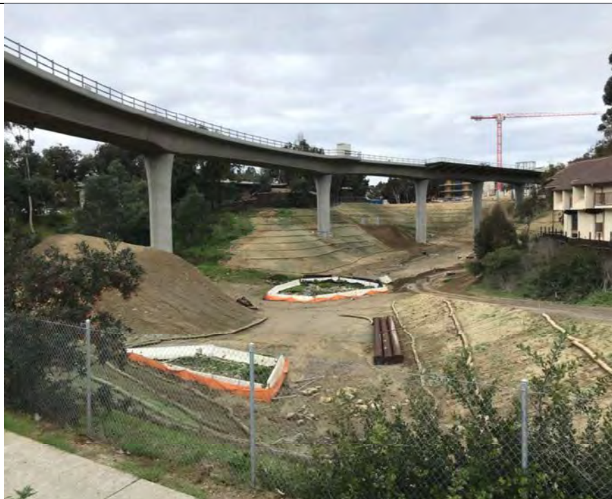
Photo 6: Current condition of NWW-1.
