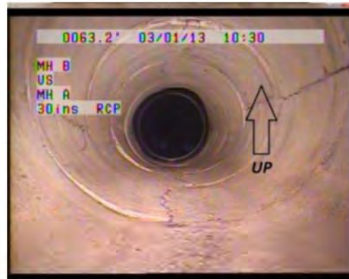
Figure 2. Longitudinal cracking in 30" RCP. This pipe is downstream of the 24" HDPE per the operator's verbal comments and survey reports, included in Appendix G.
