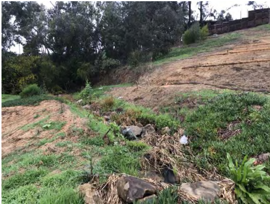
Photo 5: Current condition of NWW-1.
