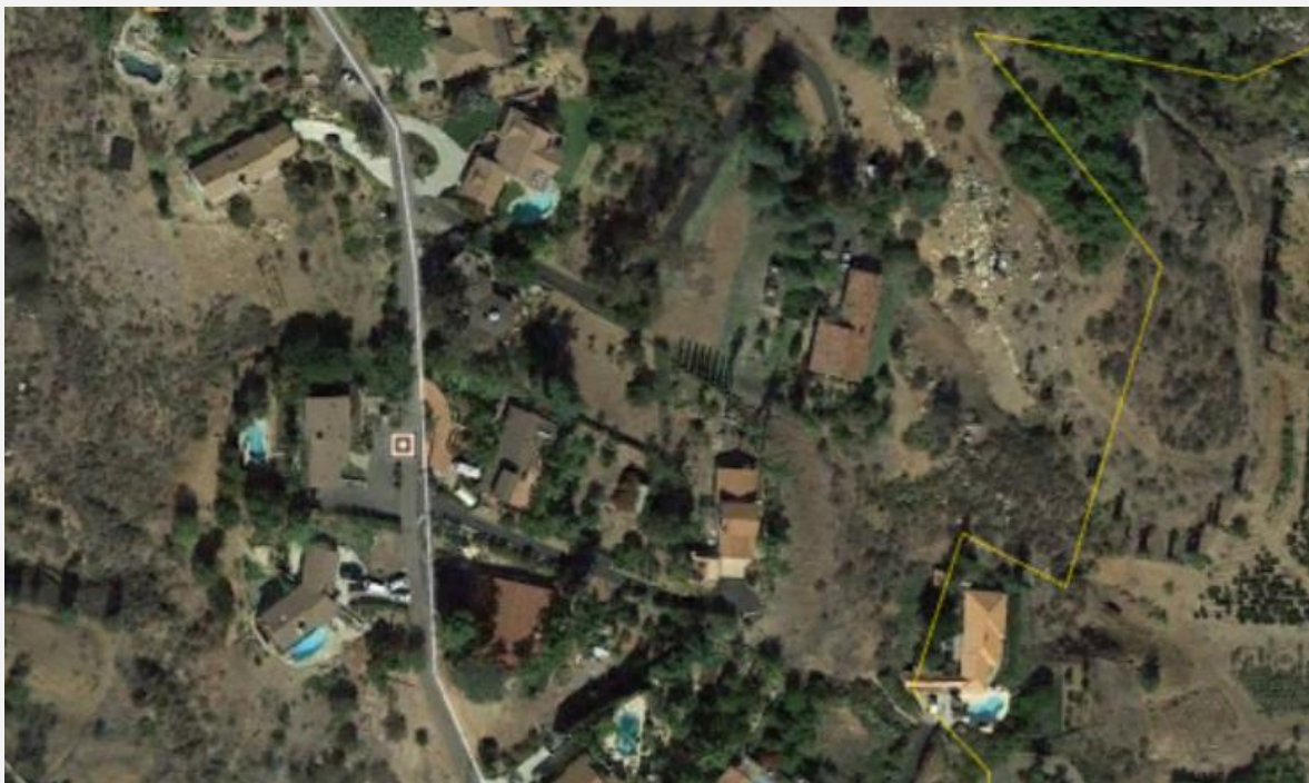
Figure 7. Example of moderate density development. Structures are located on larger properties and include varying levels of ignition resistance and landscape / fuel modification provision and maintenance. This type of development results in a higher wildland exposure level for all homes and does not provide the same buffers from wildfire encroaching onto the site, or starting at a structure and moving into the wildlands as a higher density project.
