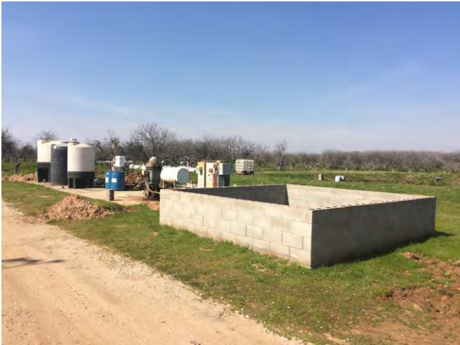
Well #3 & Storage Pond, View Facing Northwest
