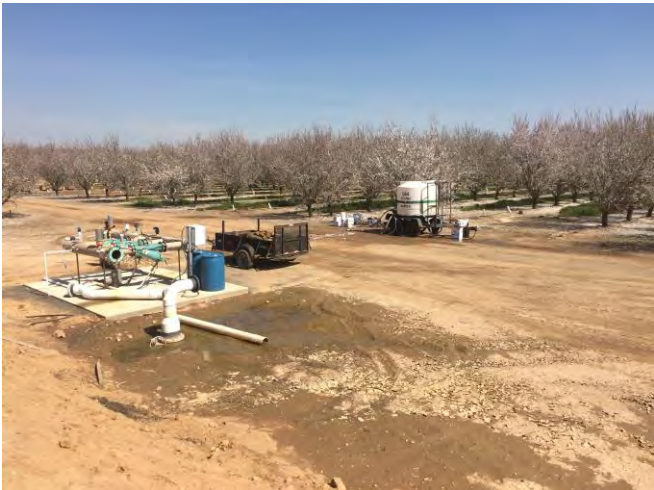
Concrete Pad East of Large Storage Pond View Facing Northeast
