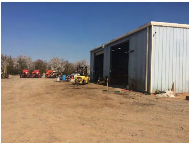
Western Side of Shop Building View Facing Northeast
