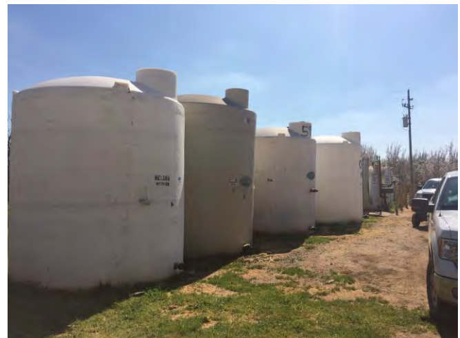
Fertilizer AST East of Shop Building View Facing Southeast
