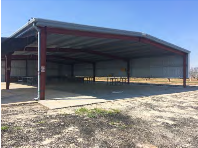
New Fruit Storage Building, View Facing Northwest
