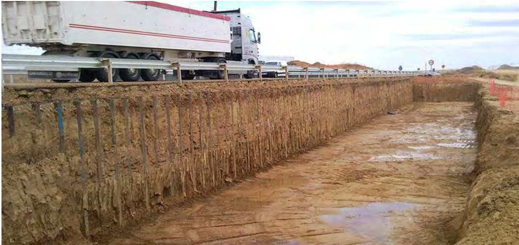
Figure 3. Wall of driven rails
