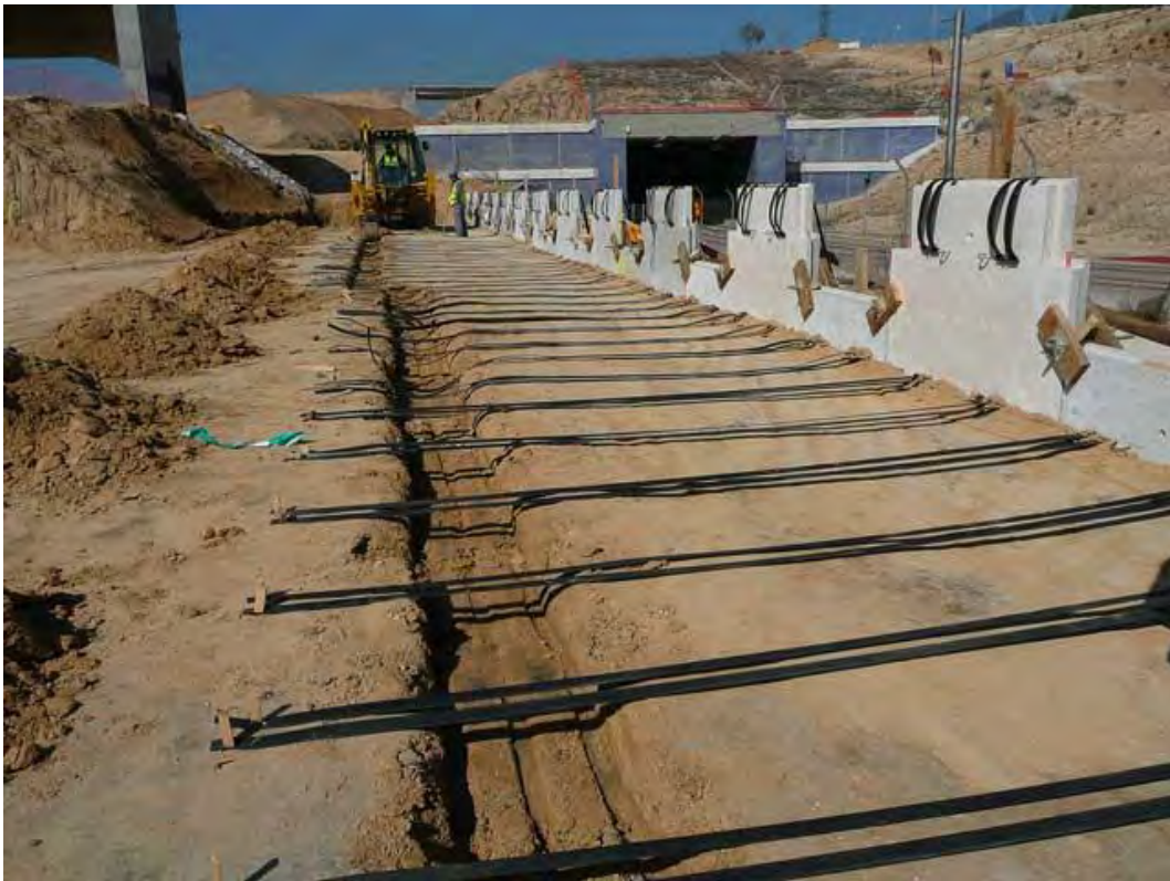
Figure 4. Reinforced earth wall execution
